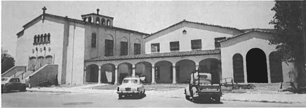
Taken Just Before Completion in 1954
