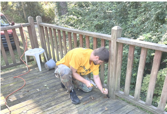
Berean James Tenny working on a deck in Spruce Pine, NC.
