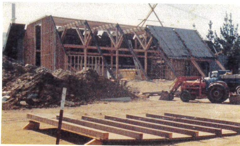
Expanding the church building in 1976, doubling its size.
