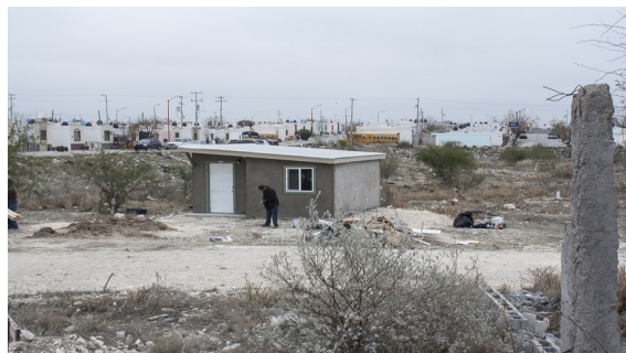
After house built
