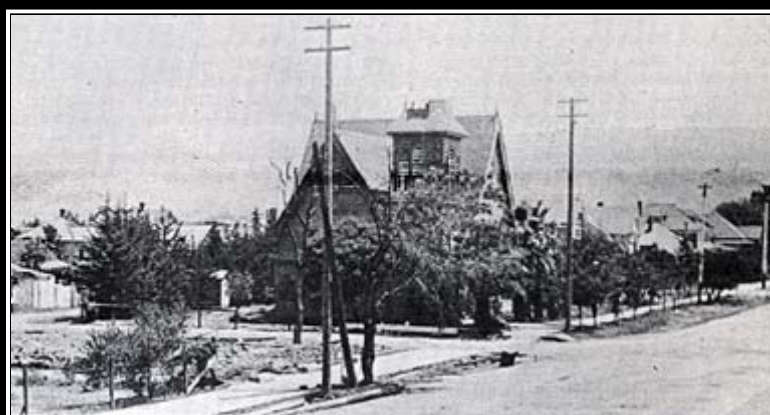
Church after steeple fire. Note that the hotel across the street is gone.
