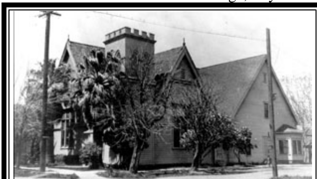
Church with the new annex complete
