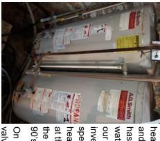
We recently discovered that the water heater on the right does not work at all and the water from the heater on the left has to go through the cold water in the water heater on the right. Which explains our lukewarm hot water. So, after some investigating, the Trustees will be spending about \$3000 on one water heater to replace them both. Take a look at the corrosion and the wet spots around the heaters. These were installed in the 90's.
