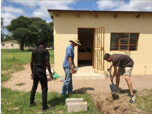
COP office and grounds preparation
