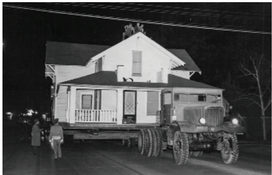
▲ Similar powerline challenges of house moving and drilling holes c1935.
