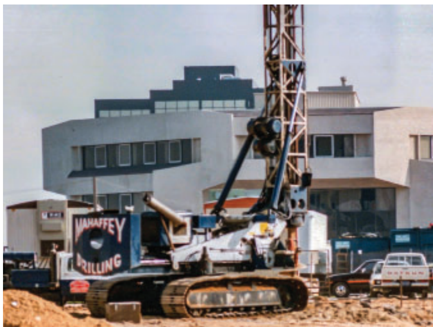
▲ 1977 2000 for ADSC member Mahaffey Drilling, another 4 th generation company.
