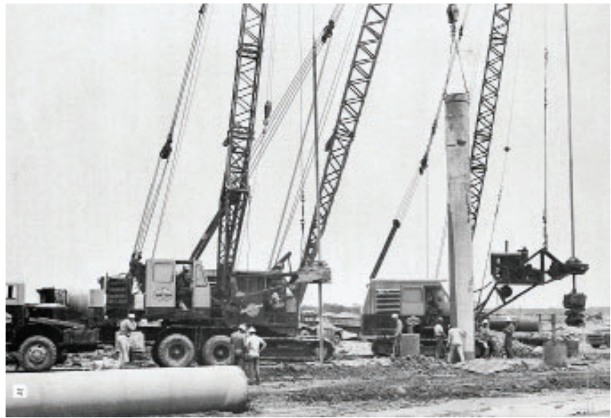
▲ 1959 Western Electric Plant, Oklahoma - 1200 60' cased piles in 90 days (Pre OSHA).
