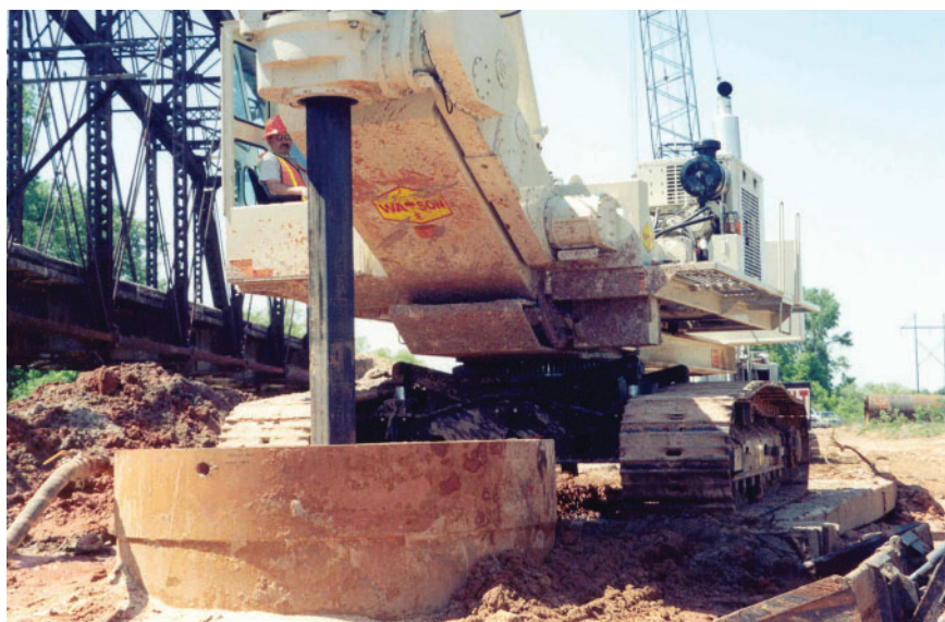
▲ Prototype 3110 built for Longfellow Drilling in 2002.
