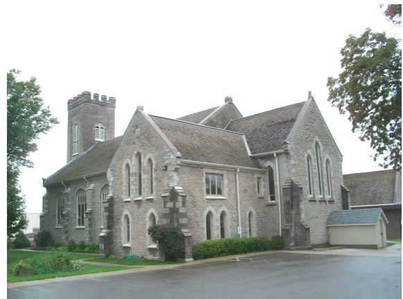
This view of the church from the Brock Street side has the vestry wing and chancel in the foreground.
