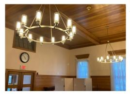
Just recently the bubs in the two chandeliers in the Chapel were changed, replacing 60-watt incandescent bulbs with 5-watt LED ones. Since 24 bubs were involved, the usage went from 1440 watts to 120, reducing the power requirement by 92%.
