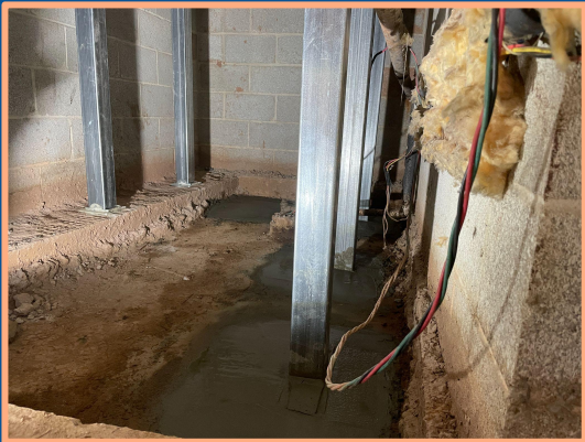
Supports in the Basement Crawlspace
