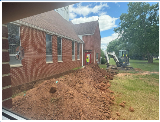
Installing Sanctuary Wall Supports
