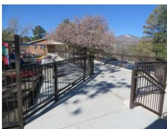
The play-lot area is almost complete. The railings that were too short to meet regulations for school yards were raised to the required 48" and bars were added at the bottom to fill in the gaps. Bondo was added to smooth the weld areas and most of the railings have been spray painted. They look very good.
