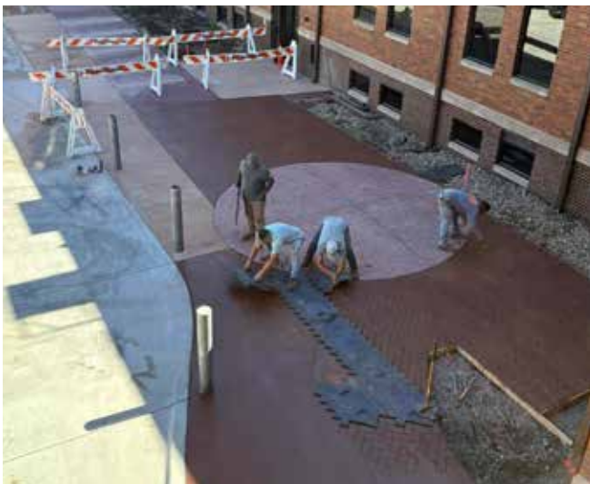
Workers made the final touches of stamping the concrete on our new entry plaza last week.
