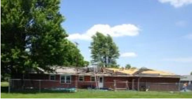
**Work began on the parsonage roof last week by J.D. Edwards Roofing and Siding of Mattoon. The roof was in bad need of re-shingling and our insurance company had denied coverage until that work was done. The cost of the roof was \$11,990.00.**
