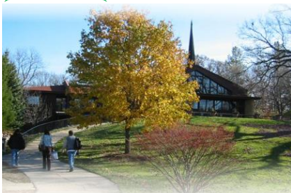
CHURCH – MAIN BUILDING
