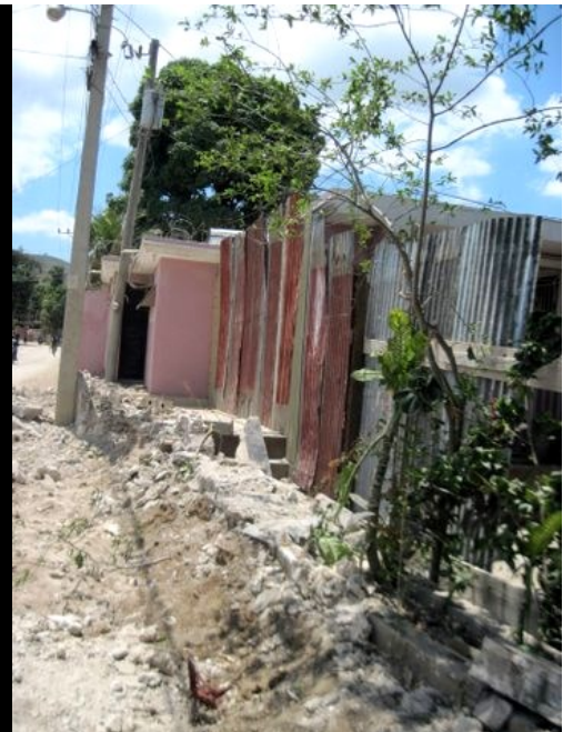
The temporary wall today!
