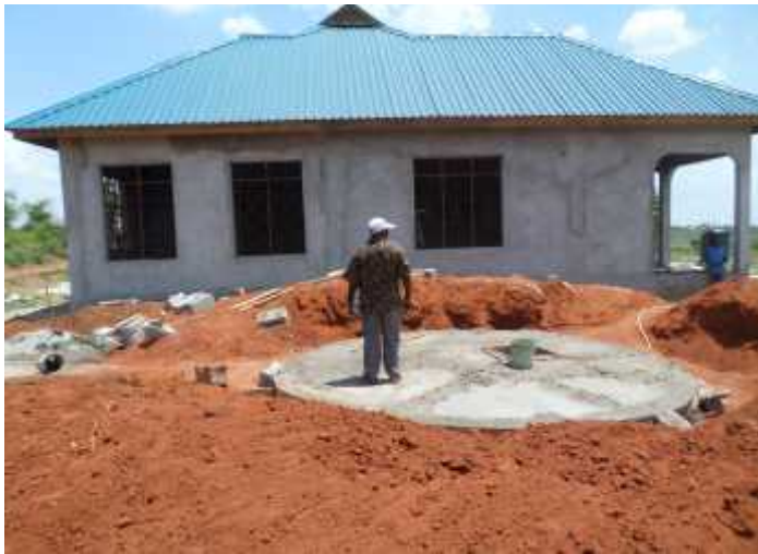
UMC Guest House Finishing, Dar es Salaam
