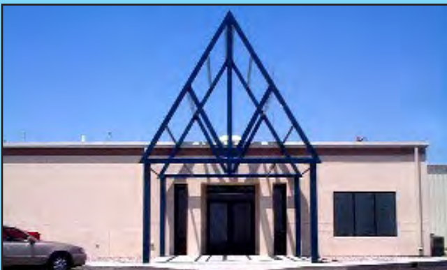
1st Phase Completed June 2001
