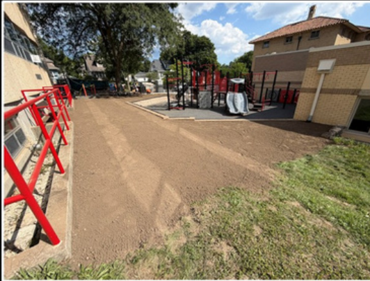
All eroded surface areas have been regraded and new topsoil placed in preparation for grass seed
