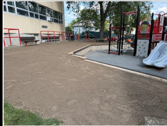
All eroded surface areas have been regraded and new topsoil placed in preparation for grass seed
