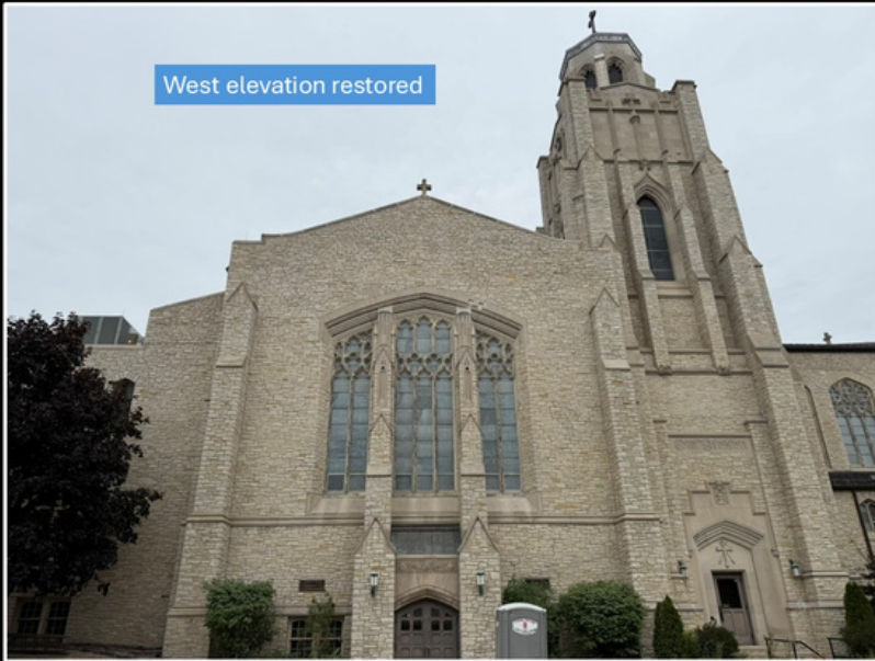
Restoration viewed from Washington Boulevard and North 55 th Street
