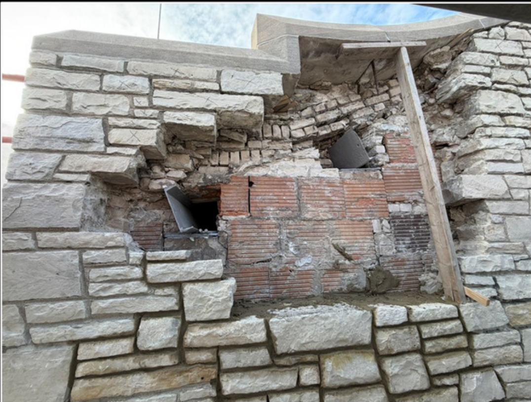
Damaged lannon stone on upper wall removed- exposing roof support beams which are in good condition
