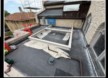
Removal of existing membrane and failed insulation on the East roof followed by installation of new insulation and rubber membrane
