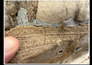
Significant deterioration of the masonry on the west gable is being addressed through partial reconstruction of wall sections, repointing of failed mortar joints and cleaning of the limestone
