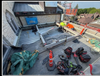
Failure of the existing roof deck structure required a new roof deck to be constructed at the West roof. Similar conditions at the SE roof will also require roof deck replacement
