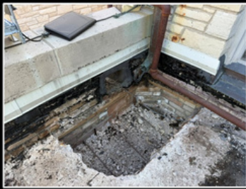
Failure of the existing roof deck structure required a new roof deck to be constructed at the West roof. Similar conditions at the SE roof will also require roof deck replacement
