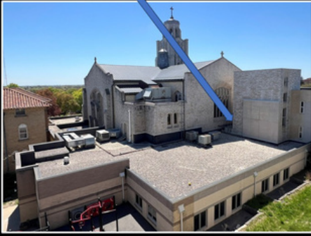
Roof area between the church and school Is being replaced
