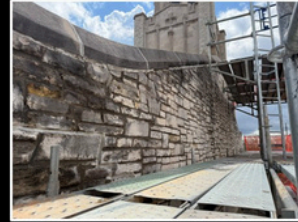
Significant deterioration of the masonry on the west gable is being addressed through partial reconstruction of wall sections, repointing of failed mortar joints and cleaning of the limestone
