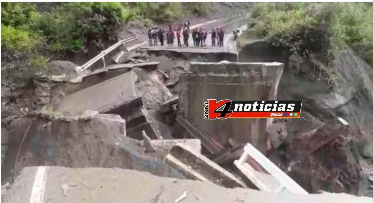
Even though this was a very well-built bridge, it couldn't stand when the accumulated water from downpours that occurred 2,000 feet above crashed into it. The other bridge a couple of miles away suffered a similar fate.
