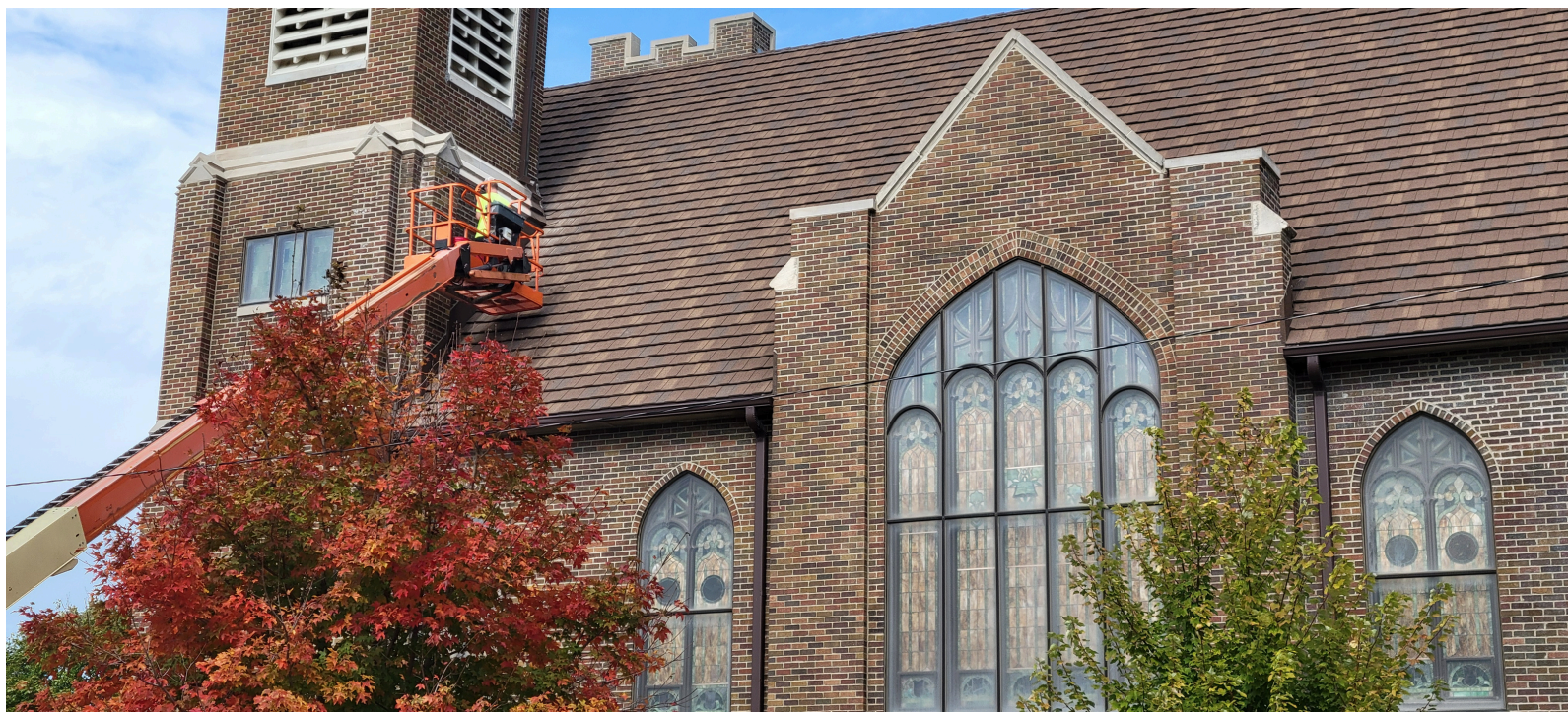
Tuckpointing on the church roof this fall.
