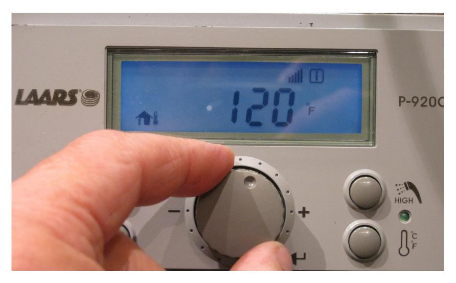
Use the Scroll/Select button and adjust to desired set point and press to lock in your selection
