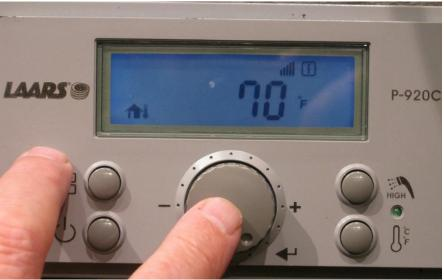
Now scroll to the desired High Out Door Temperature then press the Scroll/Select button to lock in the setting
