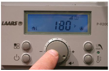
Scroll to set the desired Heating Maximum Temerature then press the Scroll/Select button to lock in
