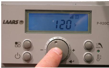
Scroll to set the desired Heating Minimum Temperature then press the Scroll/Select button to lock in
