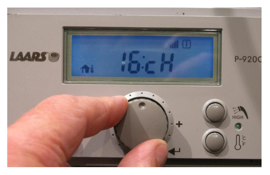
Scroll to Setting for Heating Maximum Temperature 16:cH and press Scroll/select button
