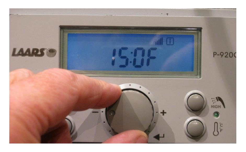
Scroll to the Warm Weather Shut Down 15:OF and press the Scroll/Select button
