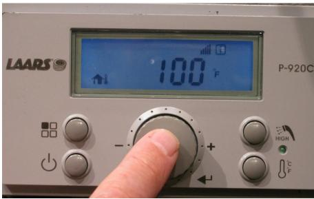
Scroll to set the desired Warm Weather Shut Down temperature then press the Scroll/Select button to lock in
