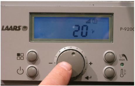
Scroll to the desired Low Out Door temperature and press the Scroll/Select button to lock in you selection
