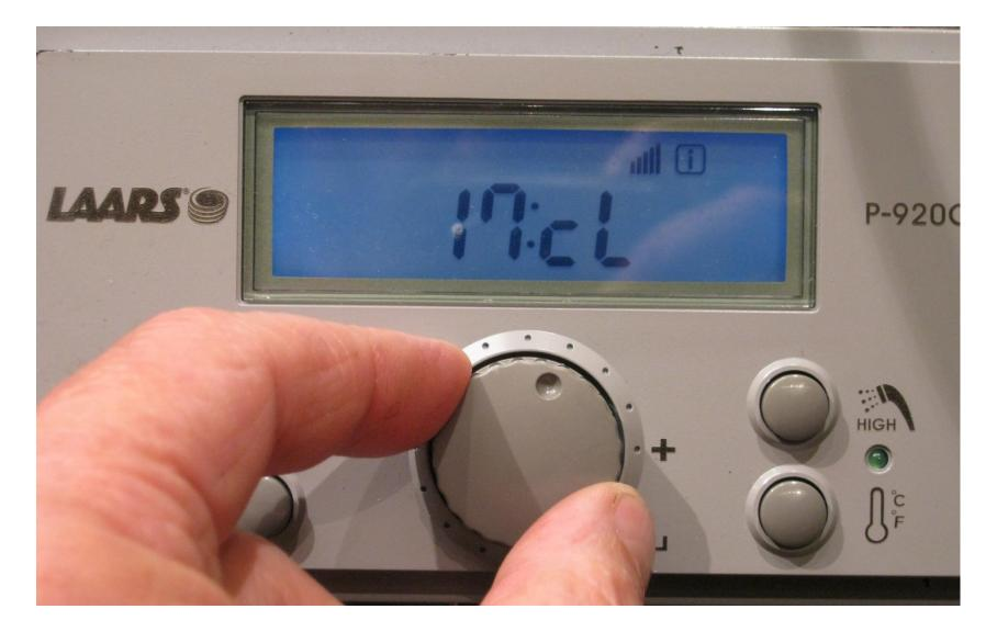
Scroll to Setting for Heating Minimum Temperature 17:cL and press Scroll/select button
