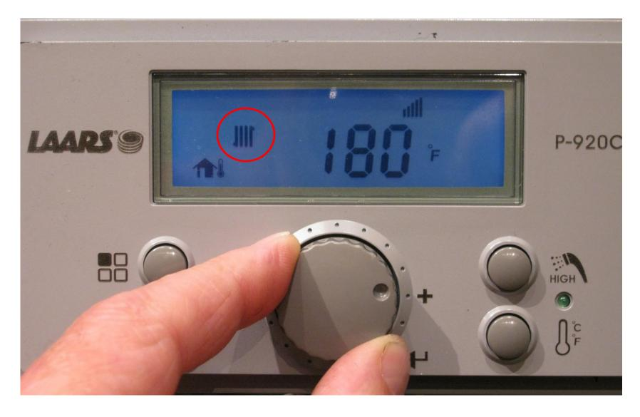
You will see the CH Icon on the screen Use the Scroll/Select button and adjust to desired set point
