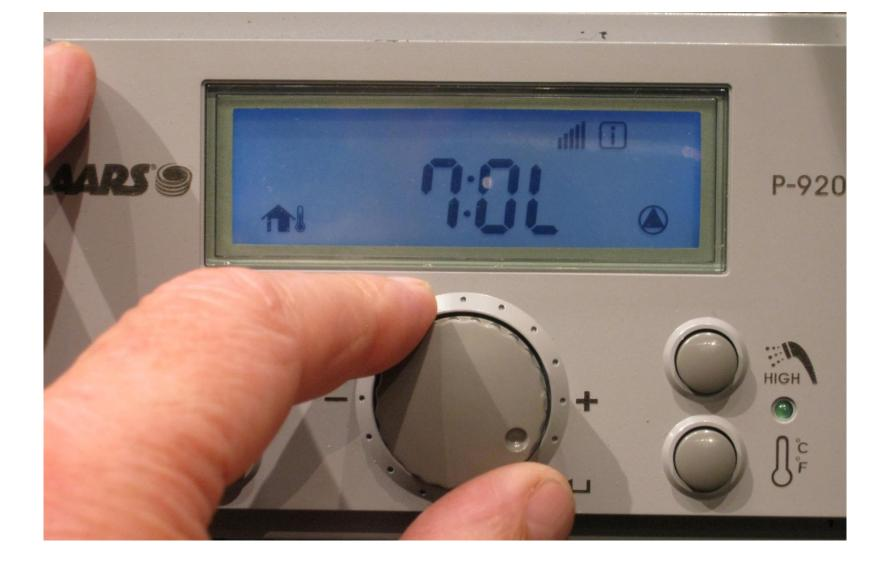
Now scroll up to 7:OL to adjust the Low Out Door temperature and press the Scroll/Select button
