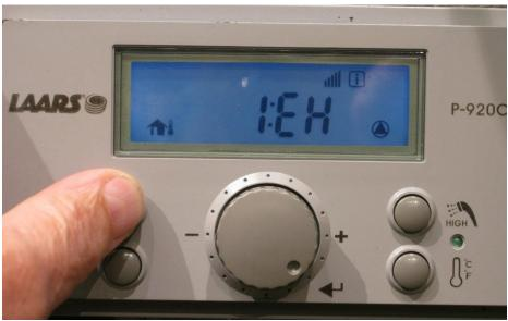
**Installer Parameters** Start by turning off the Power to the Display. Then with the Display Powered off press and HOLD the Mode button for about 5 seconds.
