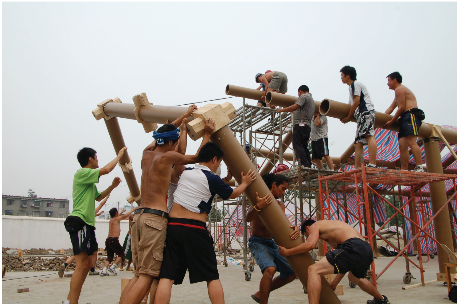
Construction of the Paper tube Arch
