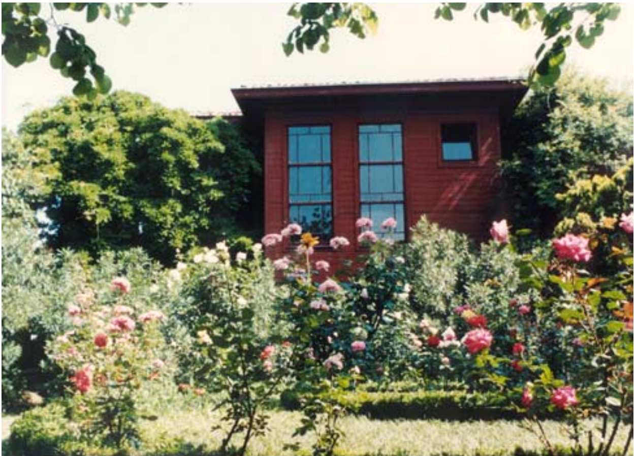
South facade, after restoration
