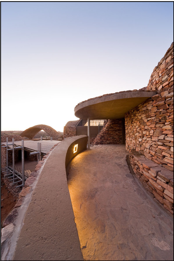
Access to the Centre is a small bridge that gives the first indication about the massing of the project.
