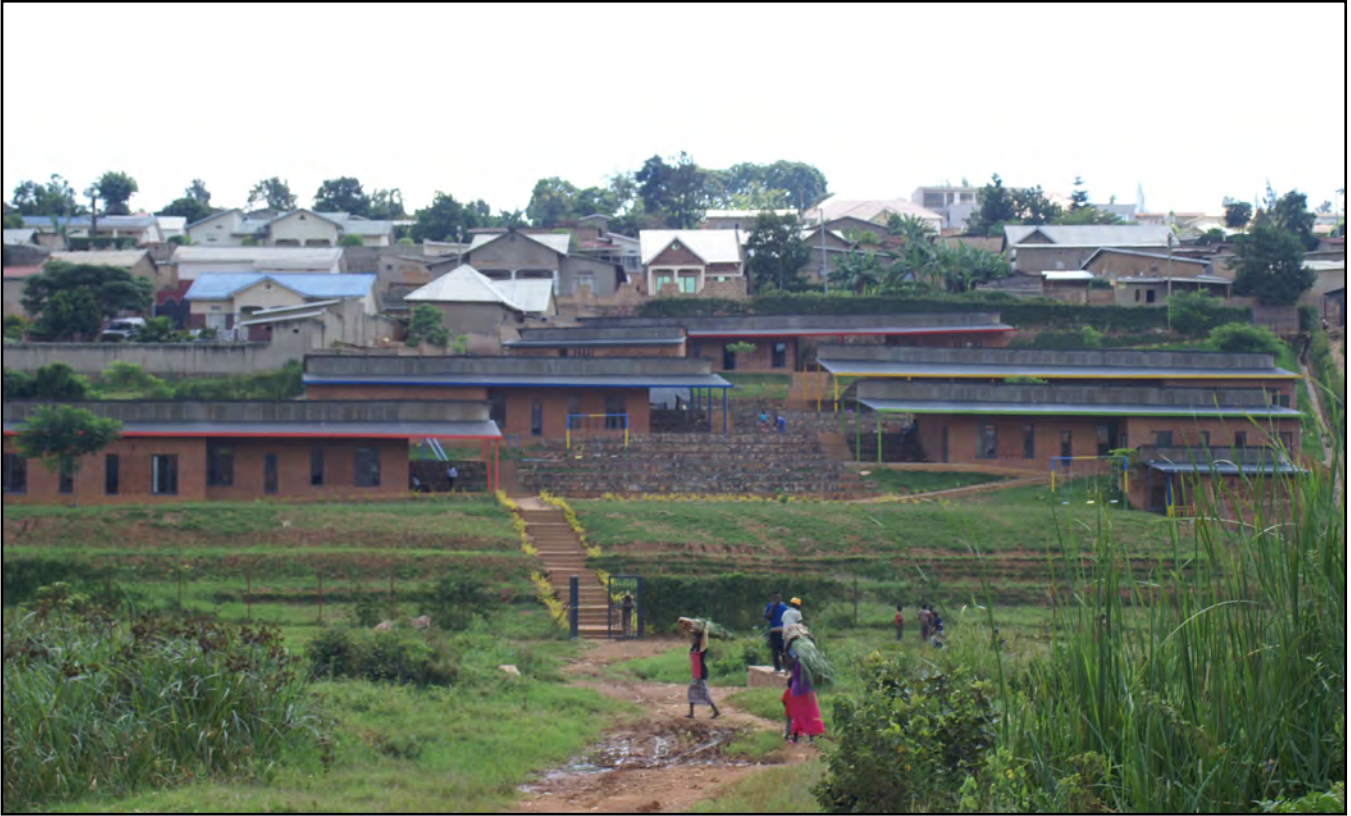
The school is built on a hillside. The slope is pretty steep so the architects had to to cope with the difficult topography. This was achieved through designing a series of platforms defining space for both the classrooms and the “courtyards” and open terraces for every age category of children.
