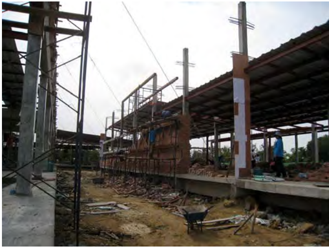
Construction start-Mock up
