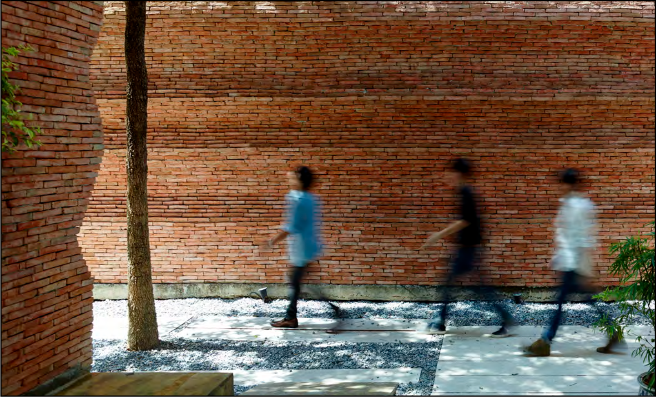
Kantana Institute uses brick to its fullest beauty. Form is of simple rectangles but the bounding walls are of undulating, double-layered brick walls that give them their very special look.
