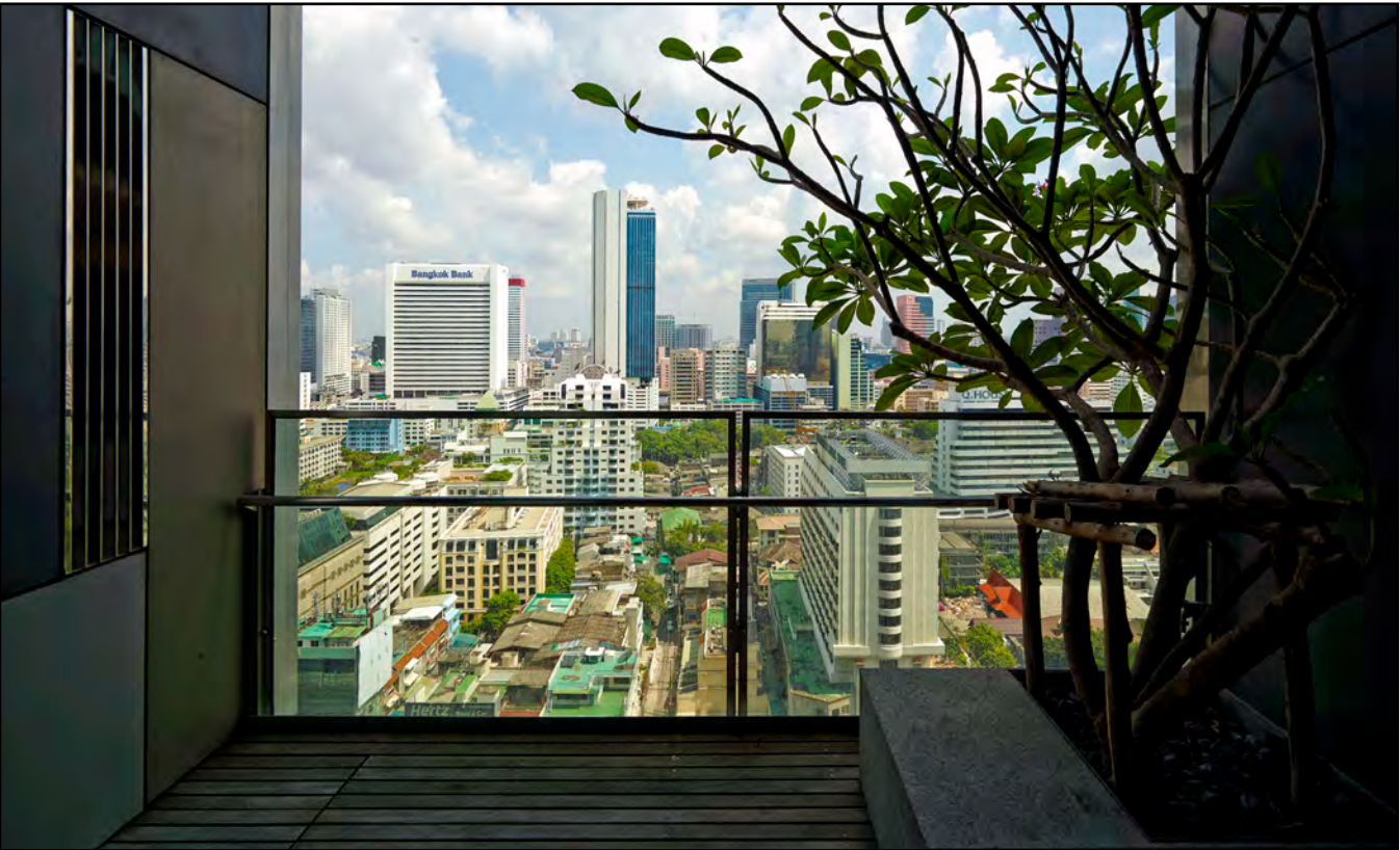
Private balconies have planters with full-sized Frangipani trees, creating almost 130% landscape ratio.
