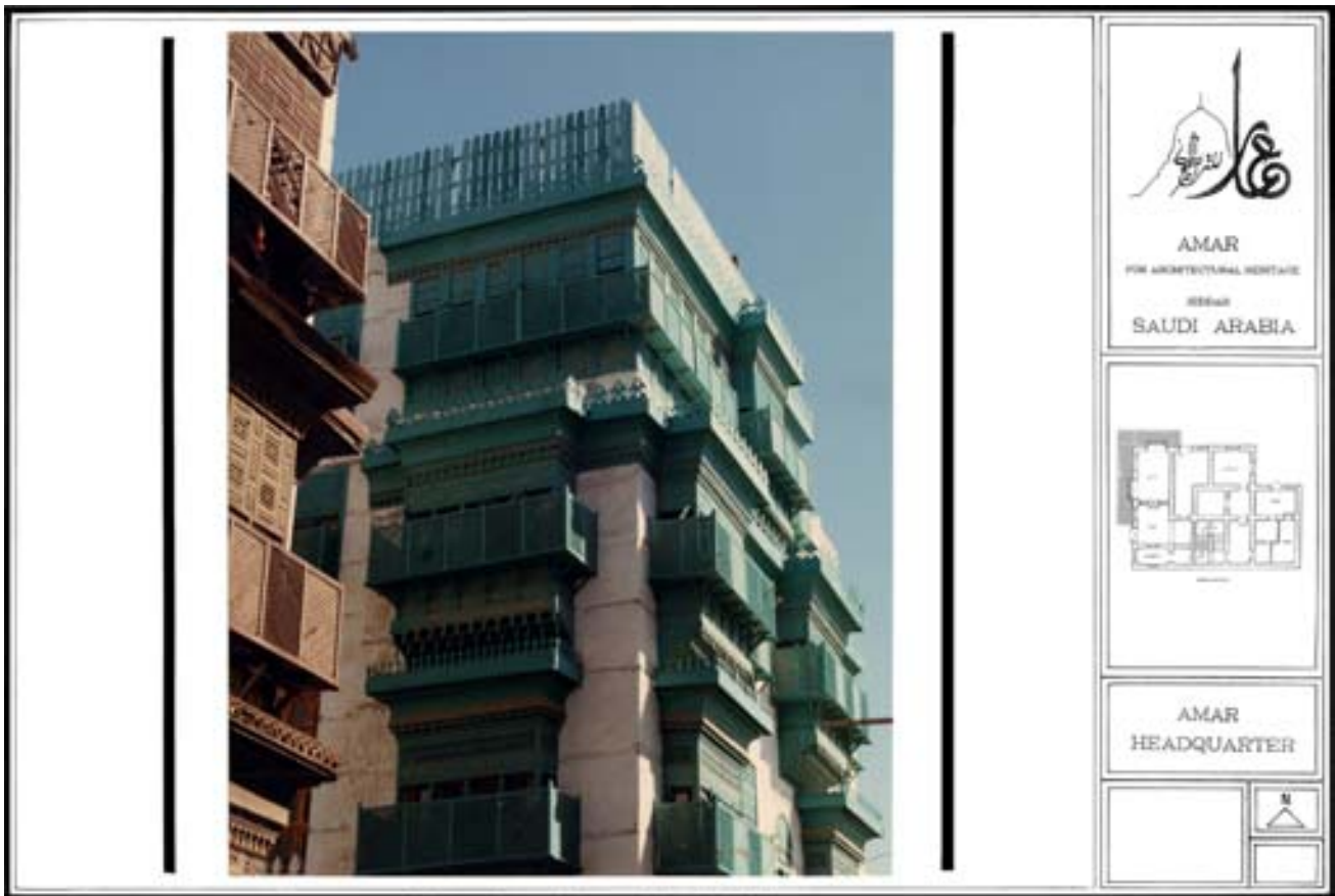
Exterior view, North-West corner
