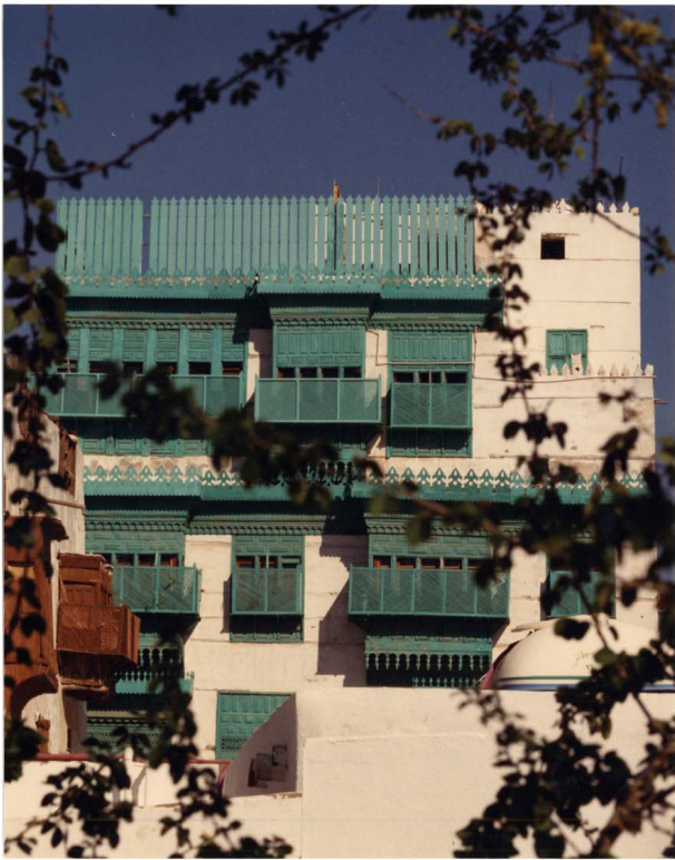
West façade, after restoration
