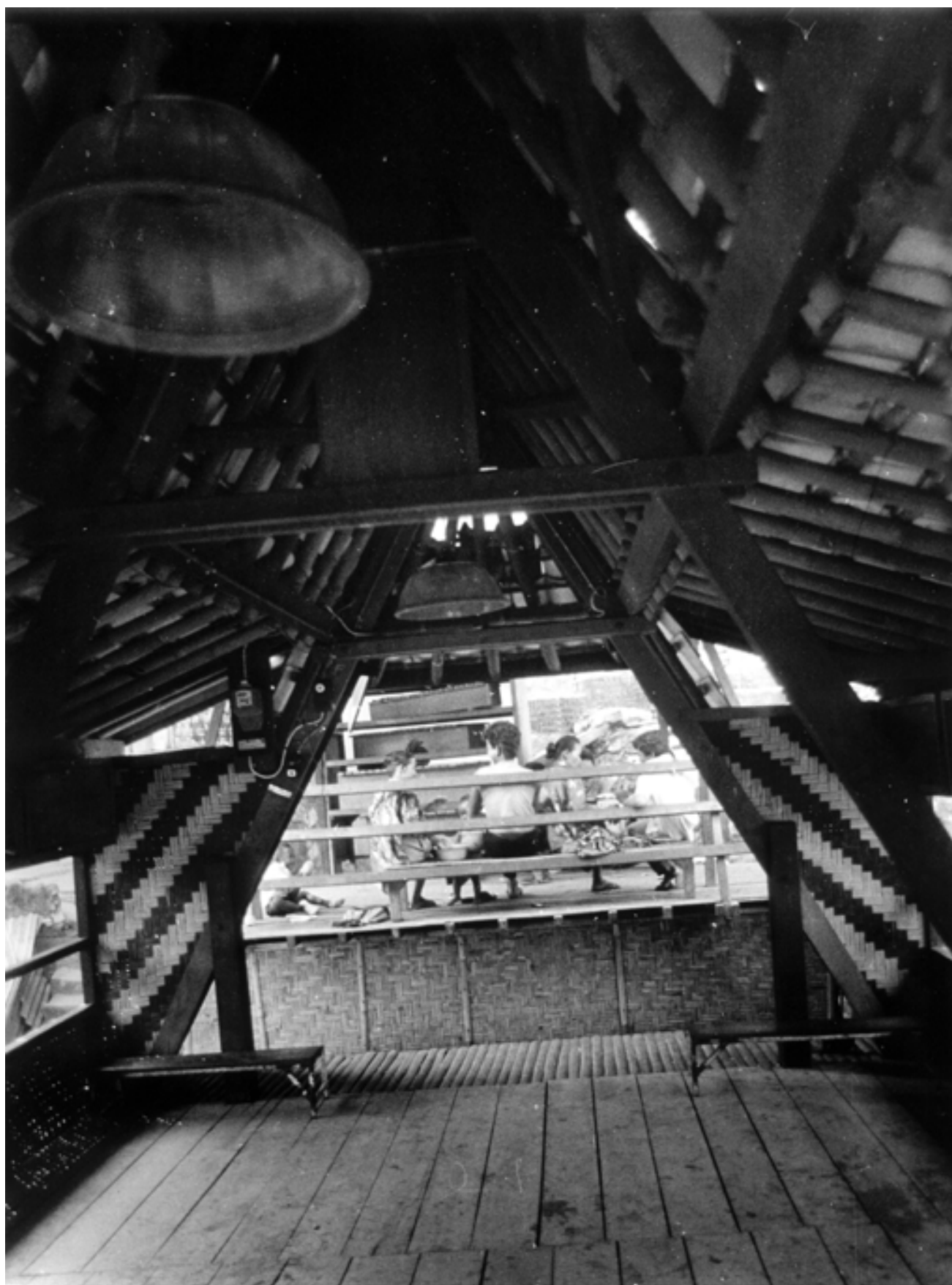
Interior, House of the Brotherhood of Neighbours, from the West
