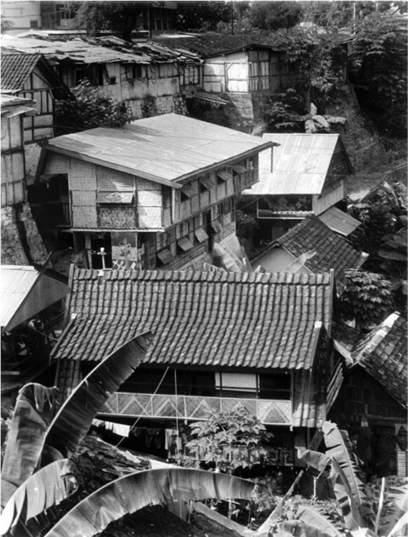
View from the North-West, detail. The building in the foreground is House of the Brotherhood of Neighbours
