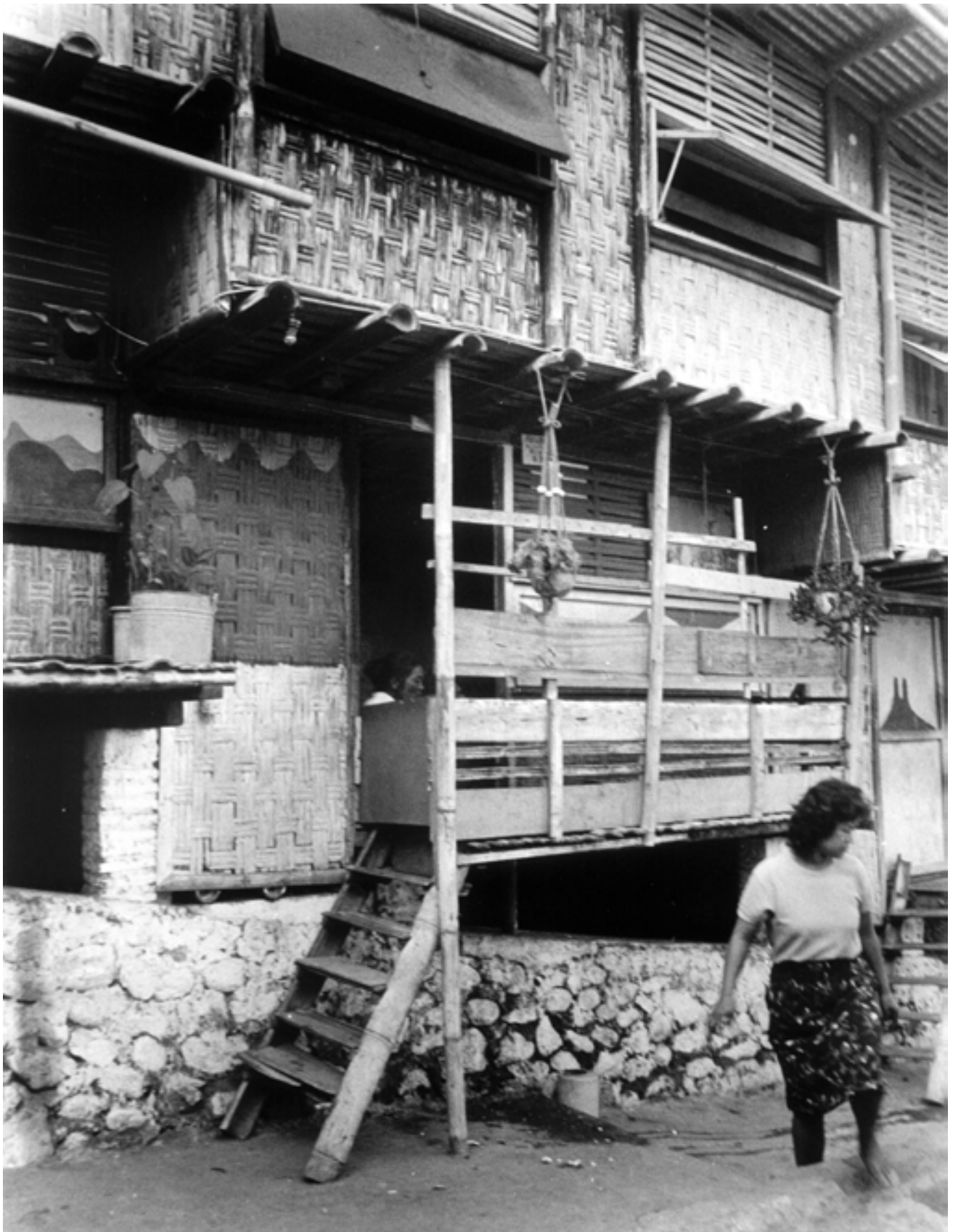
Detail of House A wall from West
