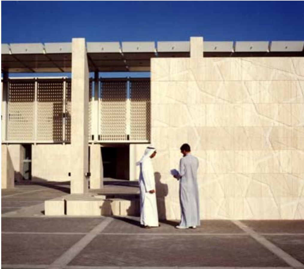
Circulation arcade and fountain stone
