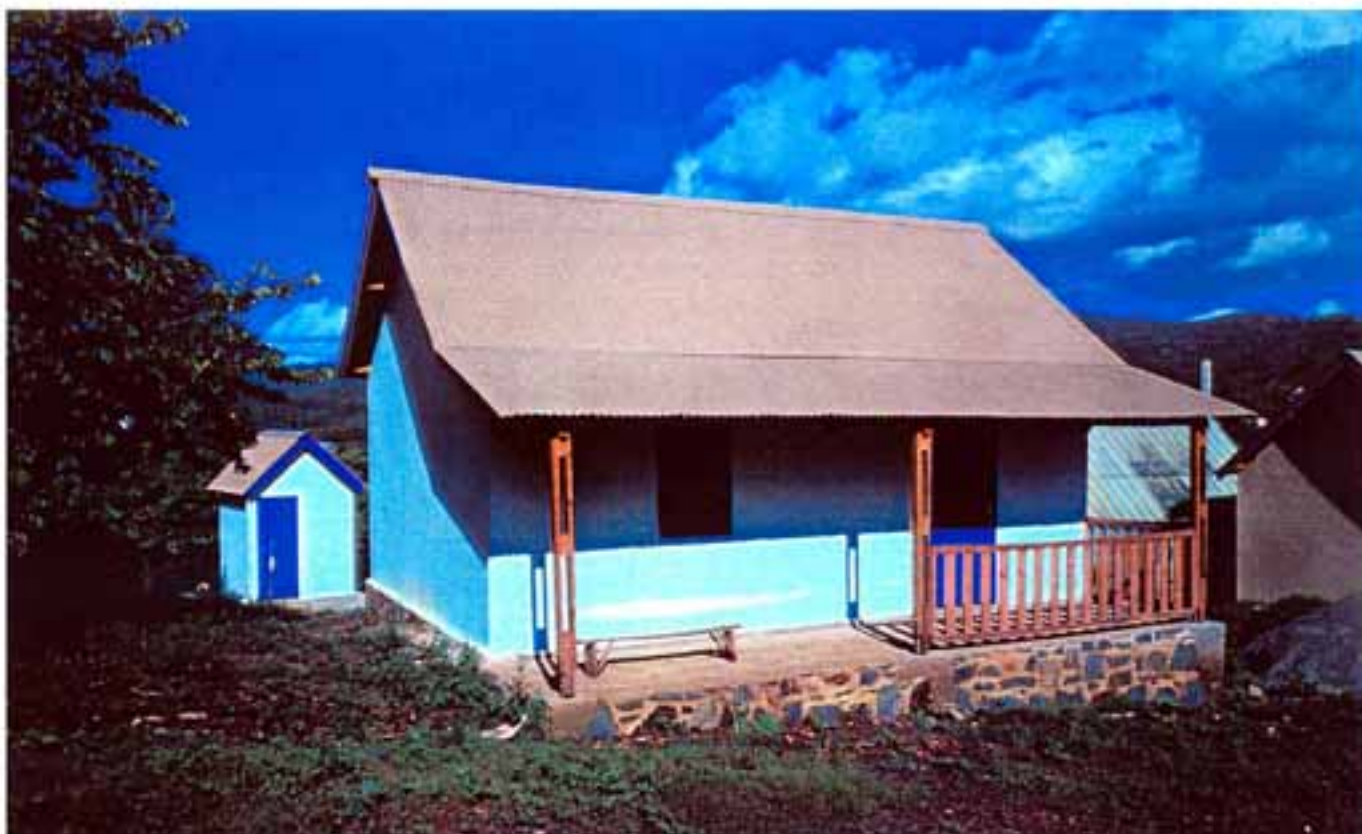
Below: The SIM architects have produced a wide variety of housing models. A typical Casé SIM unit in Chiconi has cooking facilities outside the house and a separate structure containing the toilet.
