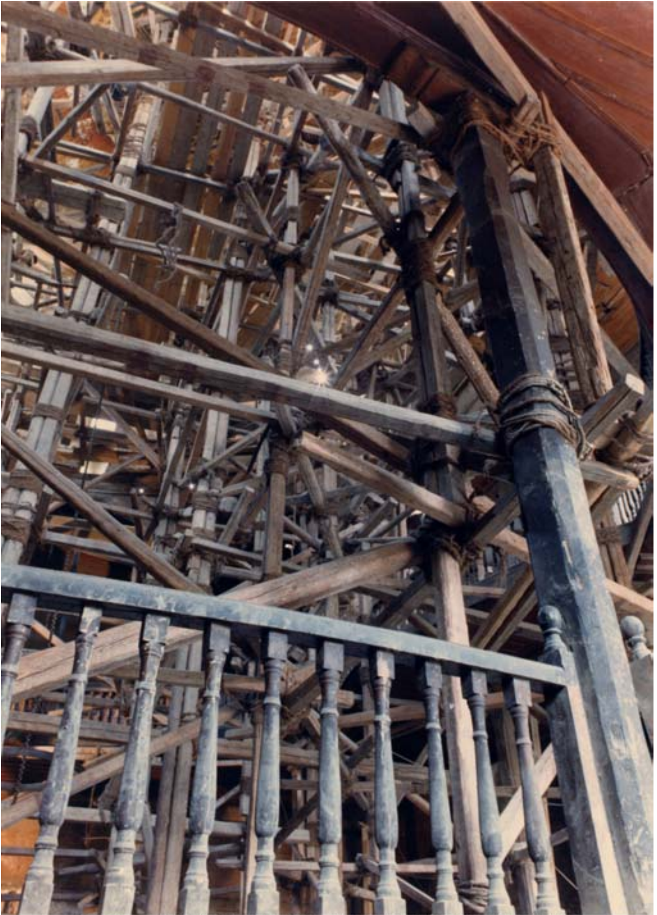
Axonometry and study of the grave statical damages of the Sama'khana: The dangerous condition has initially required an internal scaffolding made with local systems and materials in order to avoid strokes vibrations.
