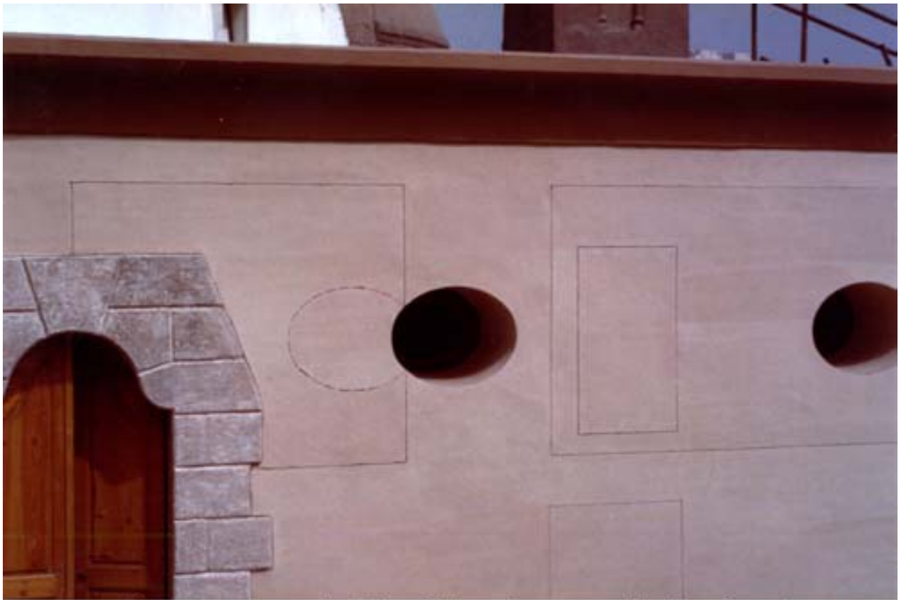
Changes and re_adaptation of the walls are graphically referred to on the finishing plaster.
