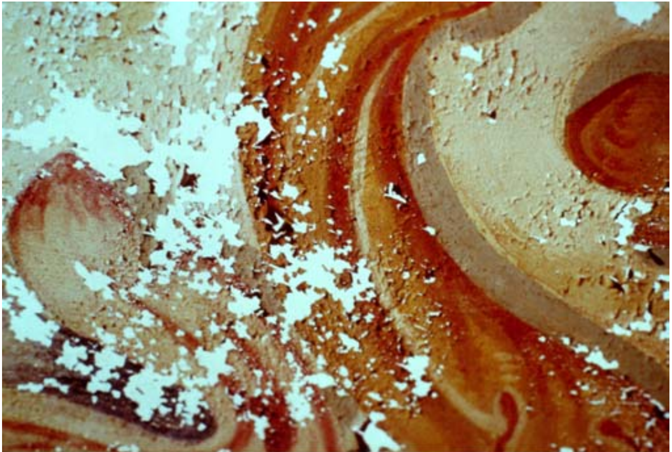
The falling flakes of the surface fixed one by one
