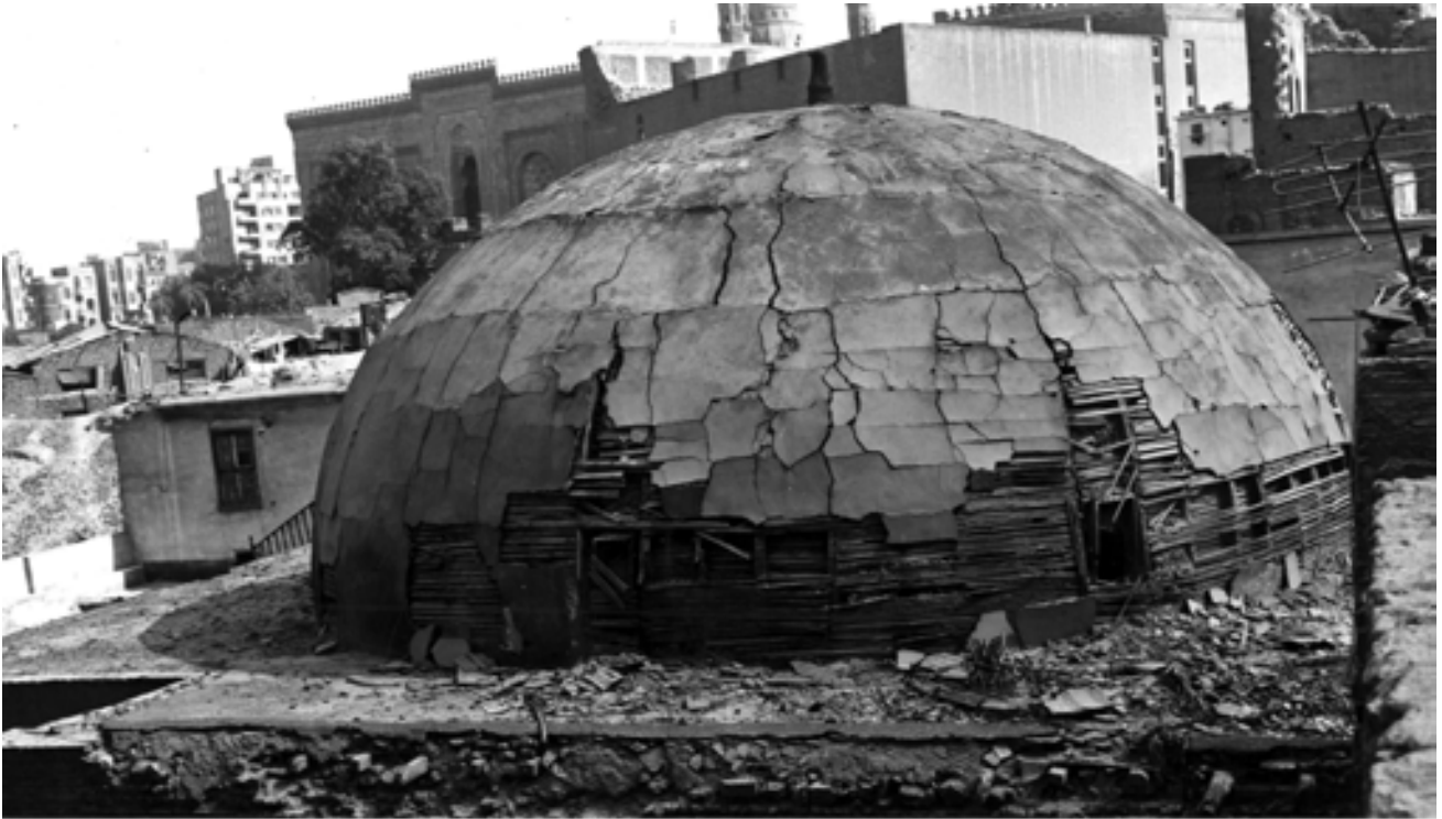
The original condition of the dome, and (at right) the initial restoration works: a system of three rings, by means of special devices and after impregnating the wood in order to restore something of its suppleness, allowed to tighten the dome and to draw it remarkably near to the primitive shape.
