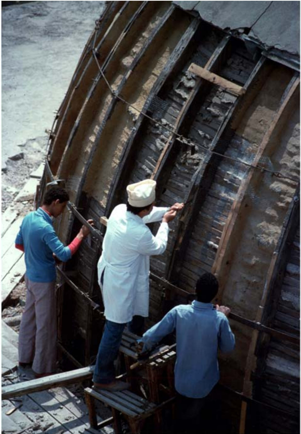
The original condition of the dome, and (at right) the initial restoration works: a system of three rings, by means of special devices and after impregnating the wood in order to restore something of its suppleness, allowed to tighten the dome and to draw it remarkably near to the primitive shape.
