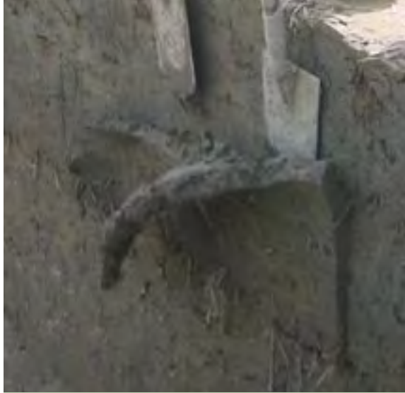
“Weller”- technique: the walls are trimmed on the sides with a spade to get the accurate shape.
