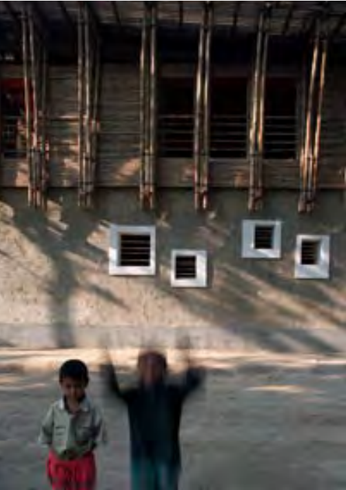
West facade, the windows got a lime plastering as rain protection.
