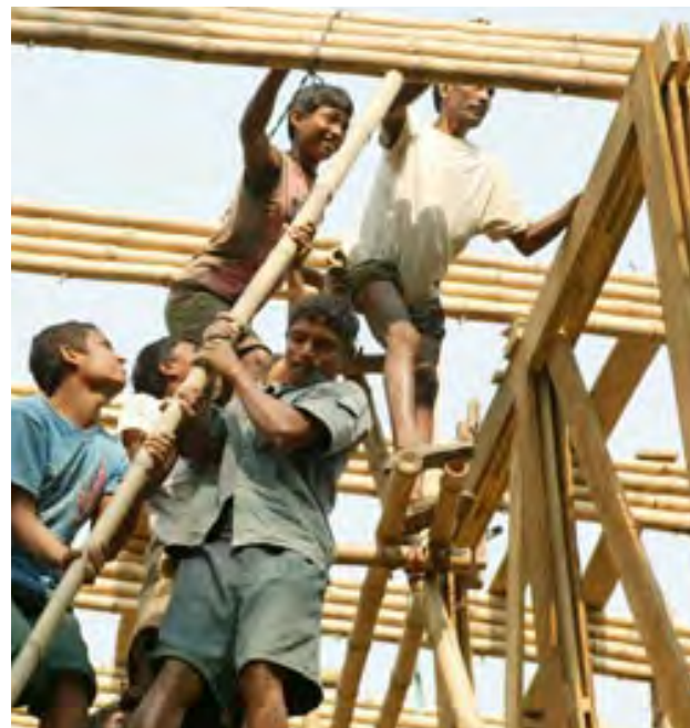
Workers fitting by hand one of 25 big bamboo frames at the 1st floor.
