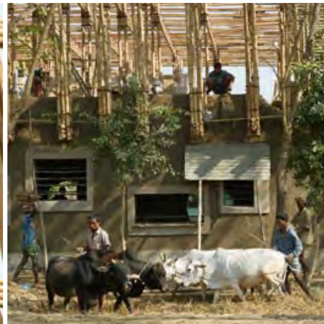
“Wireless mixing machine” - cows mixing loam and straw
