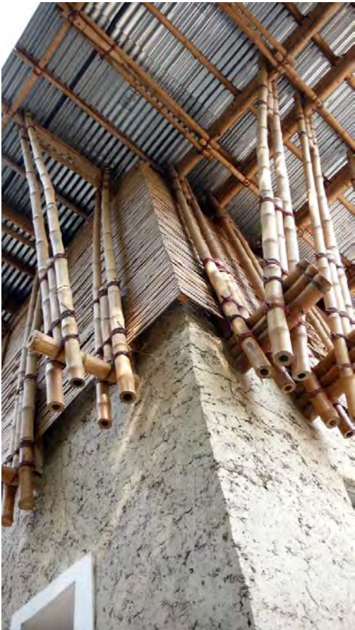
The roof is a frame construction consisting of beams - four layers of joined bamboo sticks- and vertical an diagonal poles..
