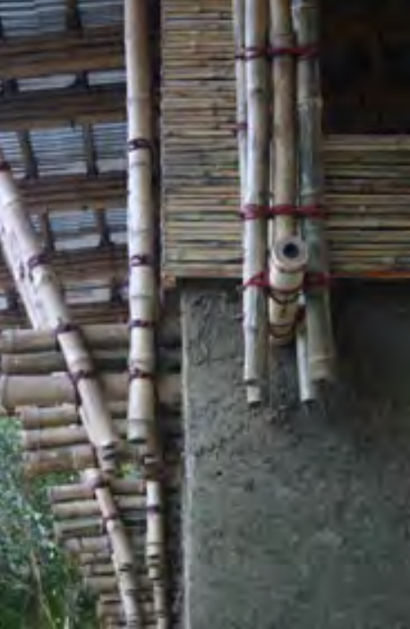
Loam wall, bamboo joints
