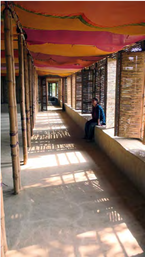
The panels, made of small bamboo sticks, provide shadow and air for a good temperature.
