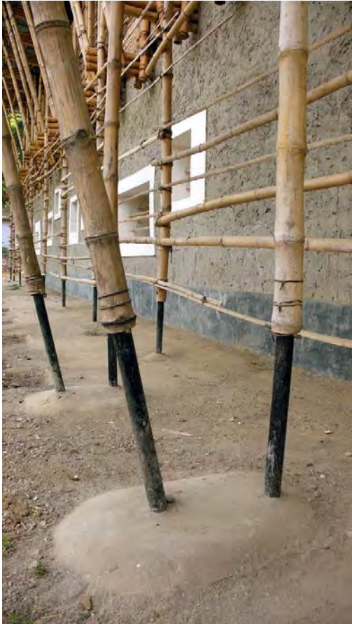
Tower supports, made of bamboo sticks.
