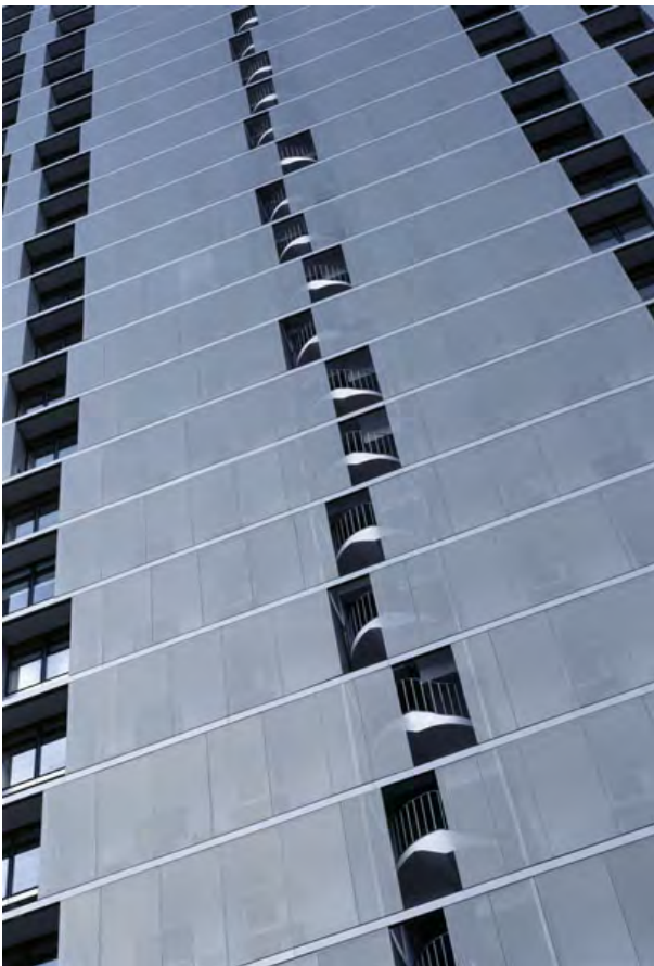
Rhythm of openings in the north façade.
