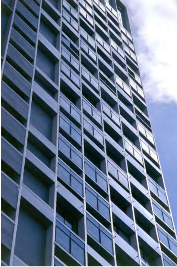
Bay windows, monsoon windows, planters and sunshades in the south façade.
