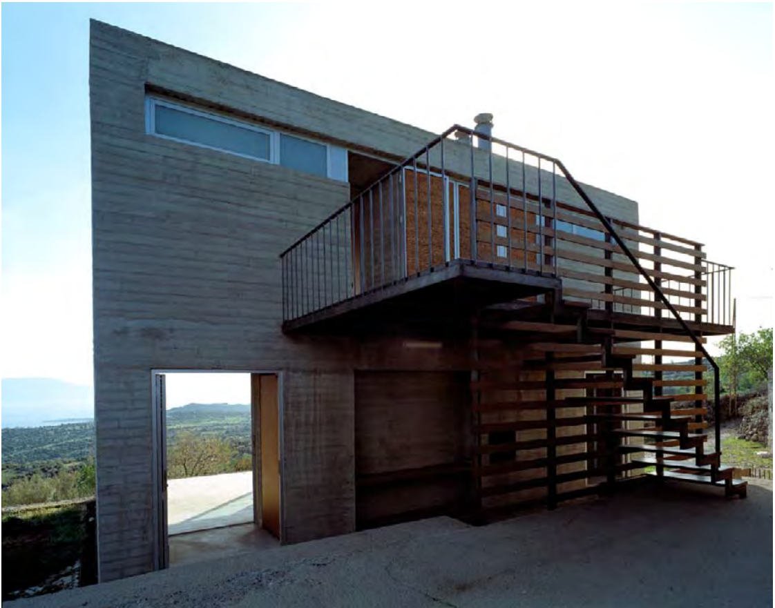
Connection between the upper and lower floors is through a light external steel framing structure with wooden planks, located at the northern façade of the building where entries to the various spaces are located.
