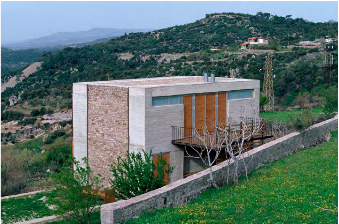
The northern façade is a 1.2-meter deep utility wall that contains most of the utilities (i.e. bathrooms, laundry space, storage, kitchenette, fireplace).
