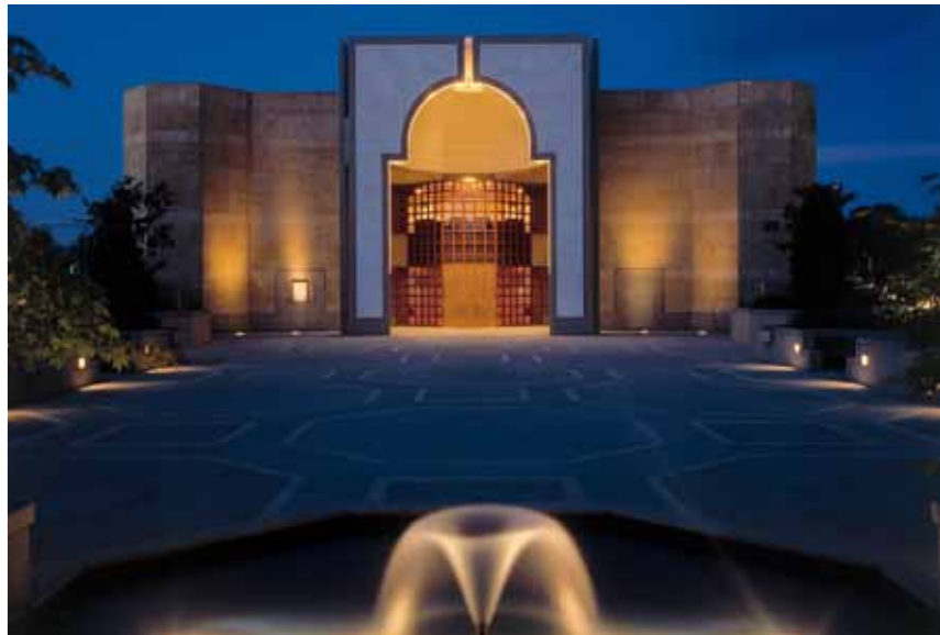
Looking past the fountain at the entrance of the Centre. The building is clad in Carrara marble and Italian sandstone. Photo: Gary Otte
