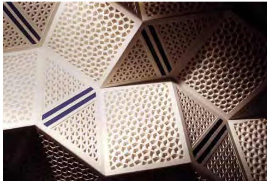
The honey comb ceiling (muqarnas) designed by Karl Schlamminger is a relief seeking design that gives a sense of greater height.
