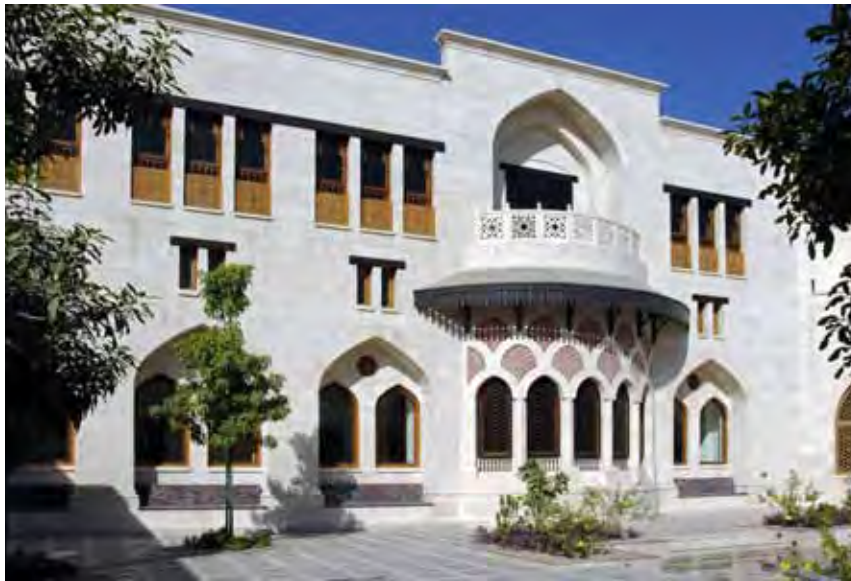
A façade of interspersed openings facing the courtyard
