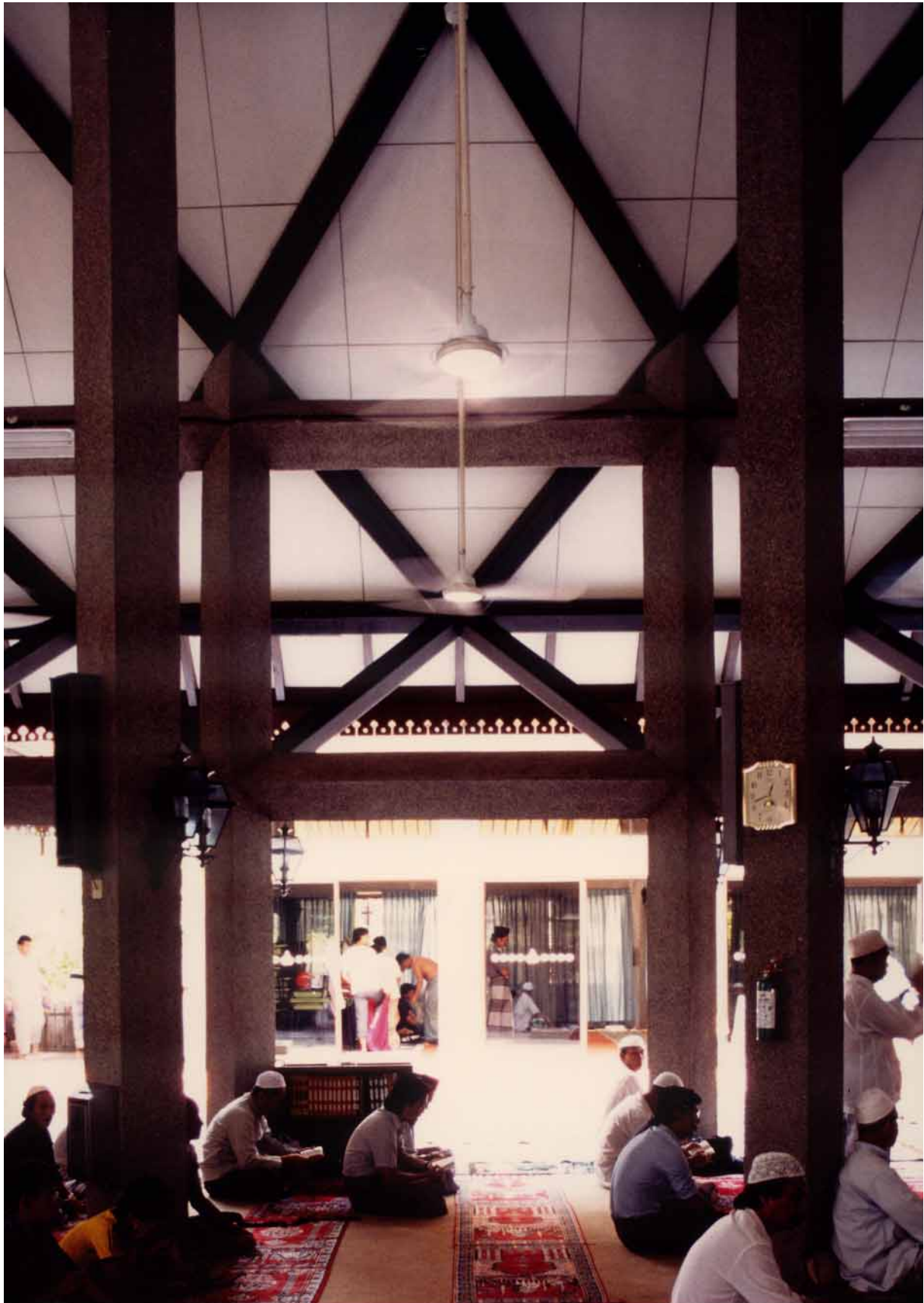
High extended prayer hall with deep roof overhang creating a cool, ventilated space
