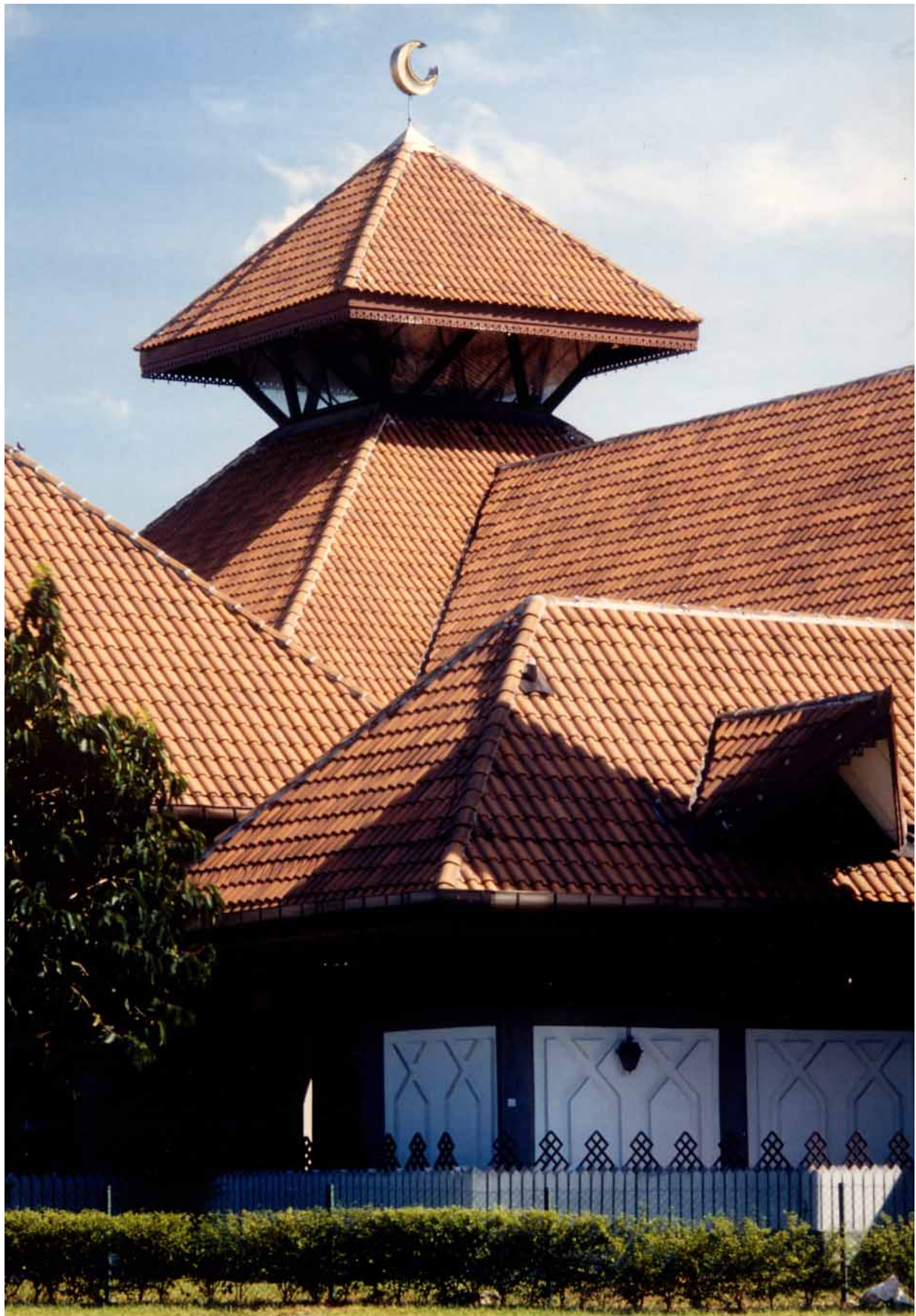
Partial view of elevation
