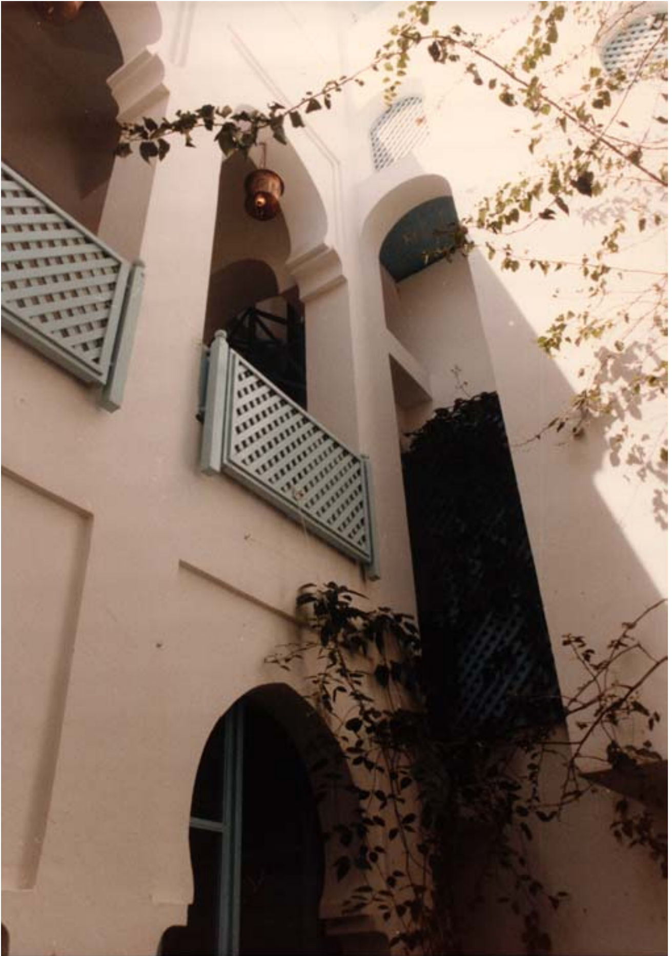
View of internal Patio from below with wooden mashrabiyyas used as Gallery's Parapets
