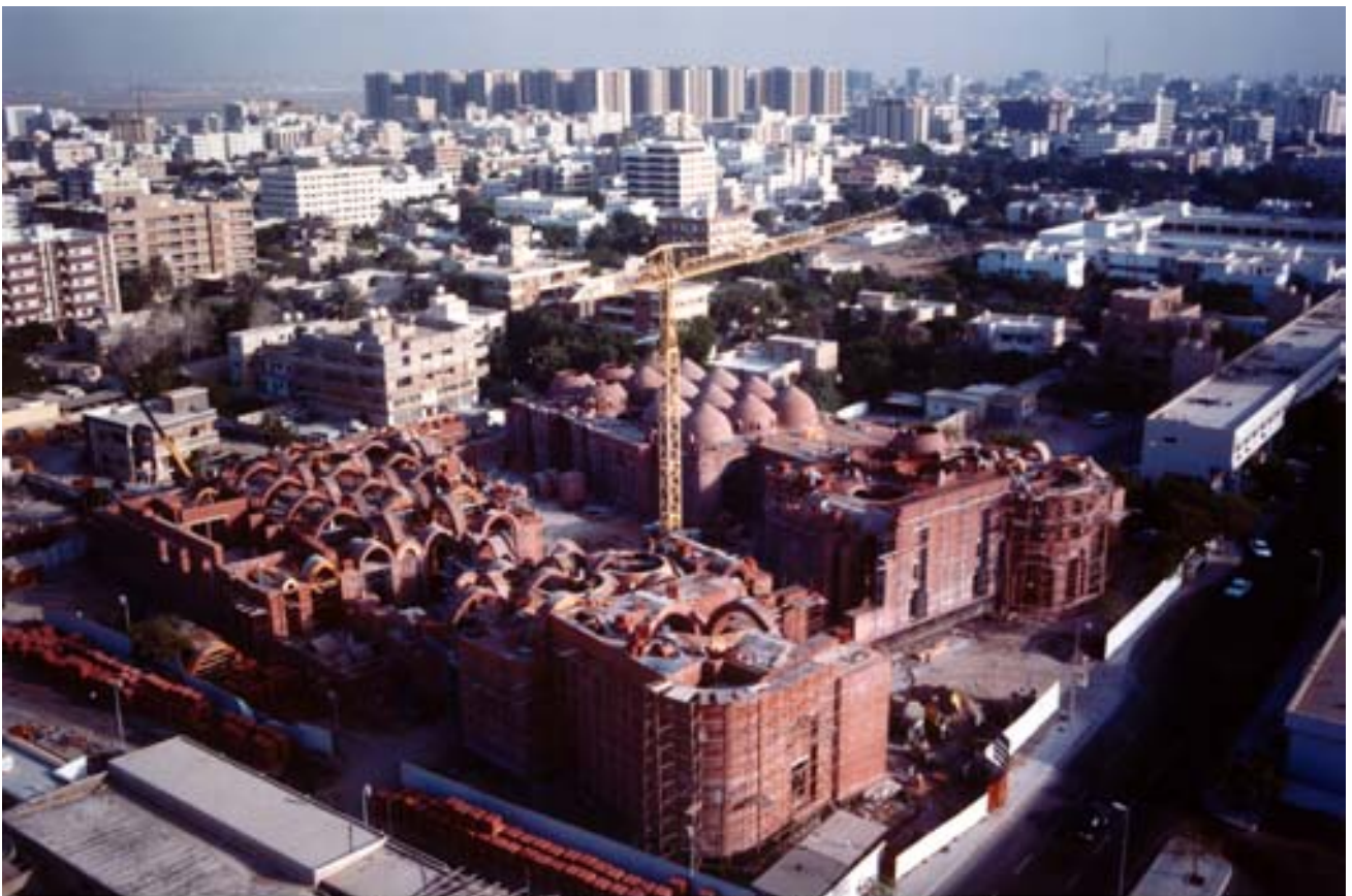
King Saud Mosque during Construction
