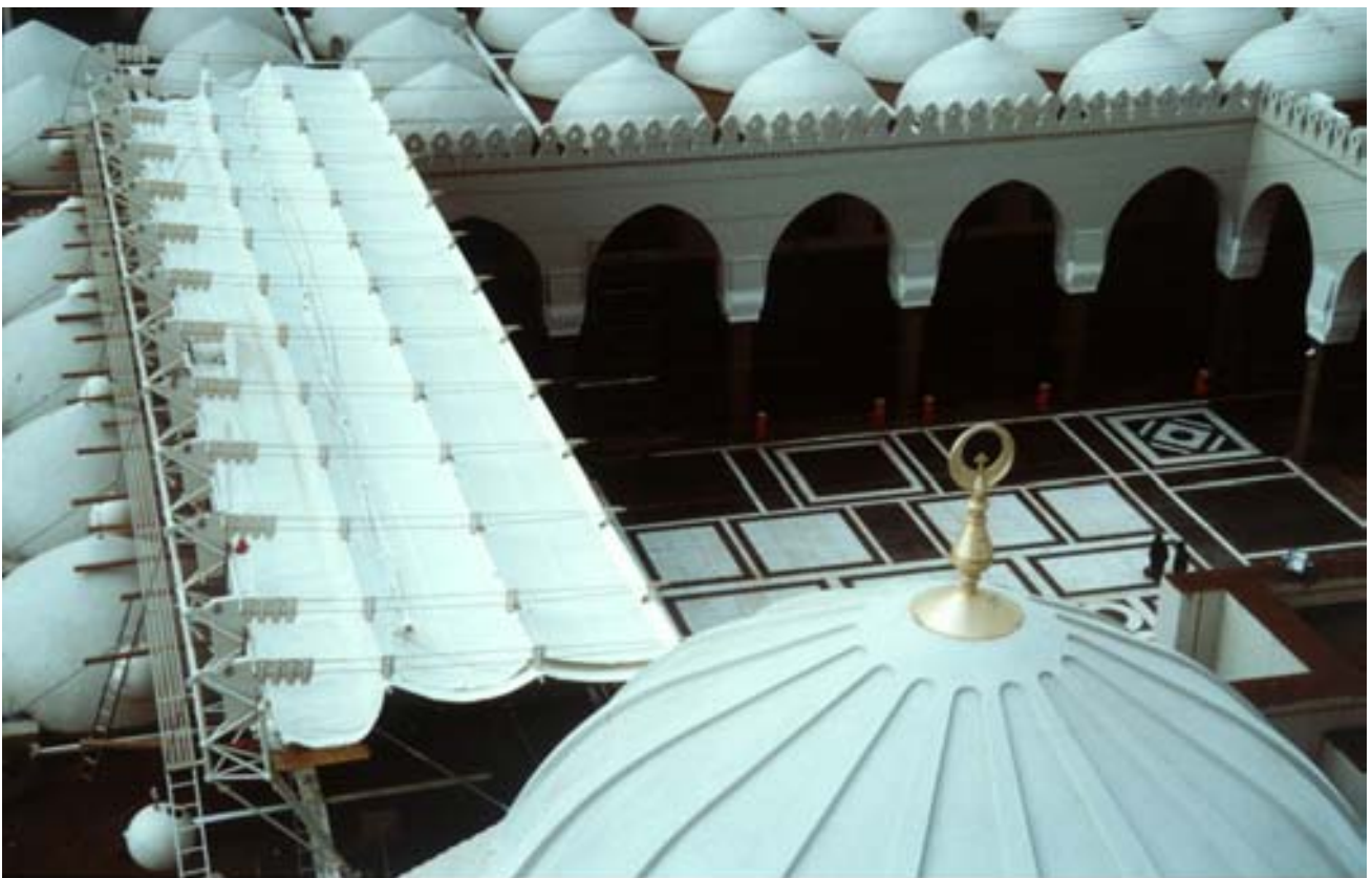
Qubba Mosque: Motorized Pulleys Closing the Tent over the Courtyard
