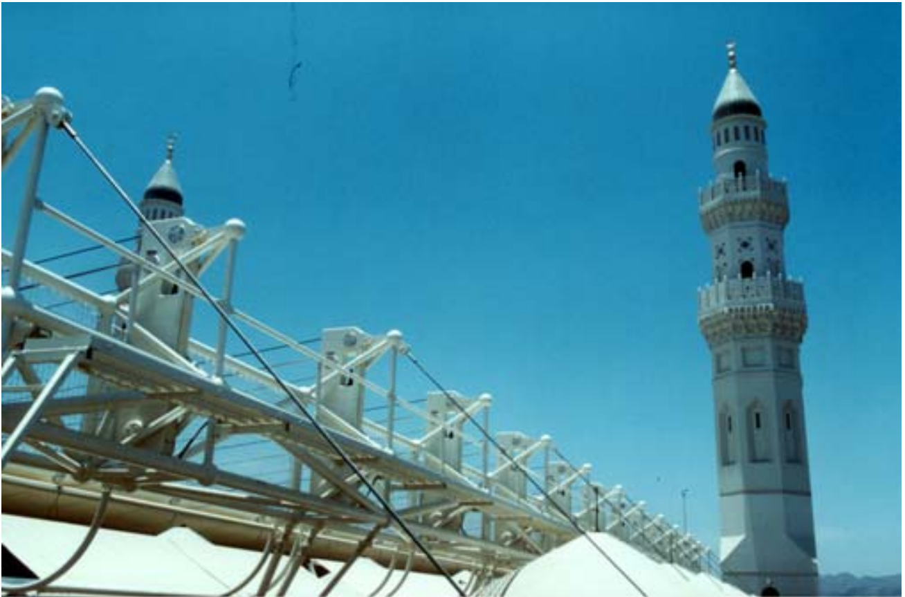
Qubba Mosque: Detail of retractable Tent Construction
