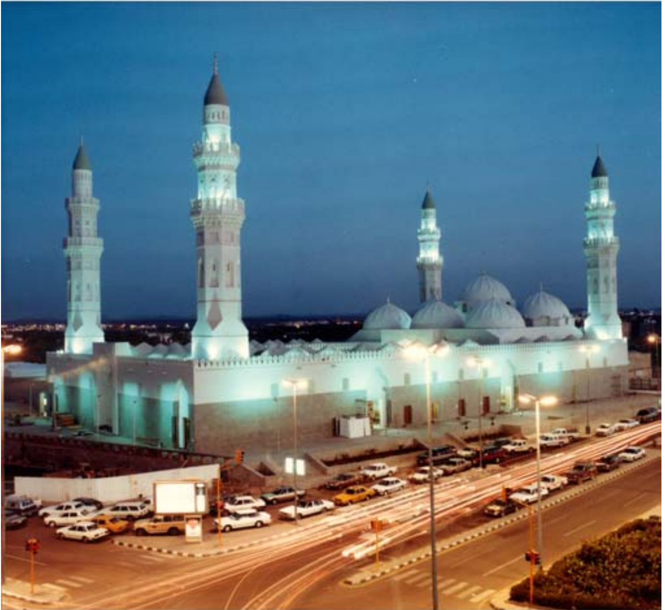
Qubba Mosque: Overall View and Access Roads
