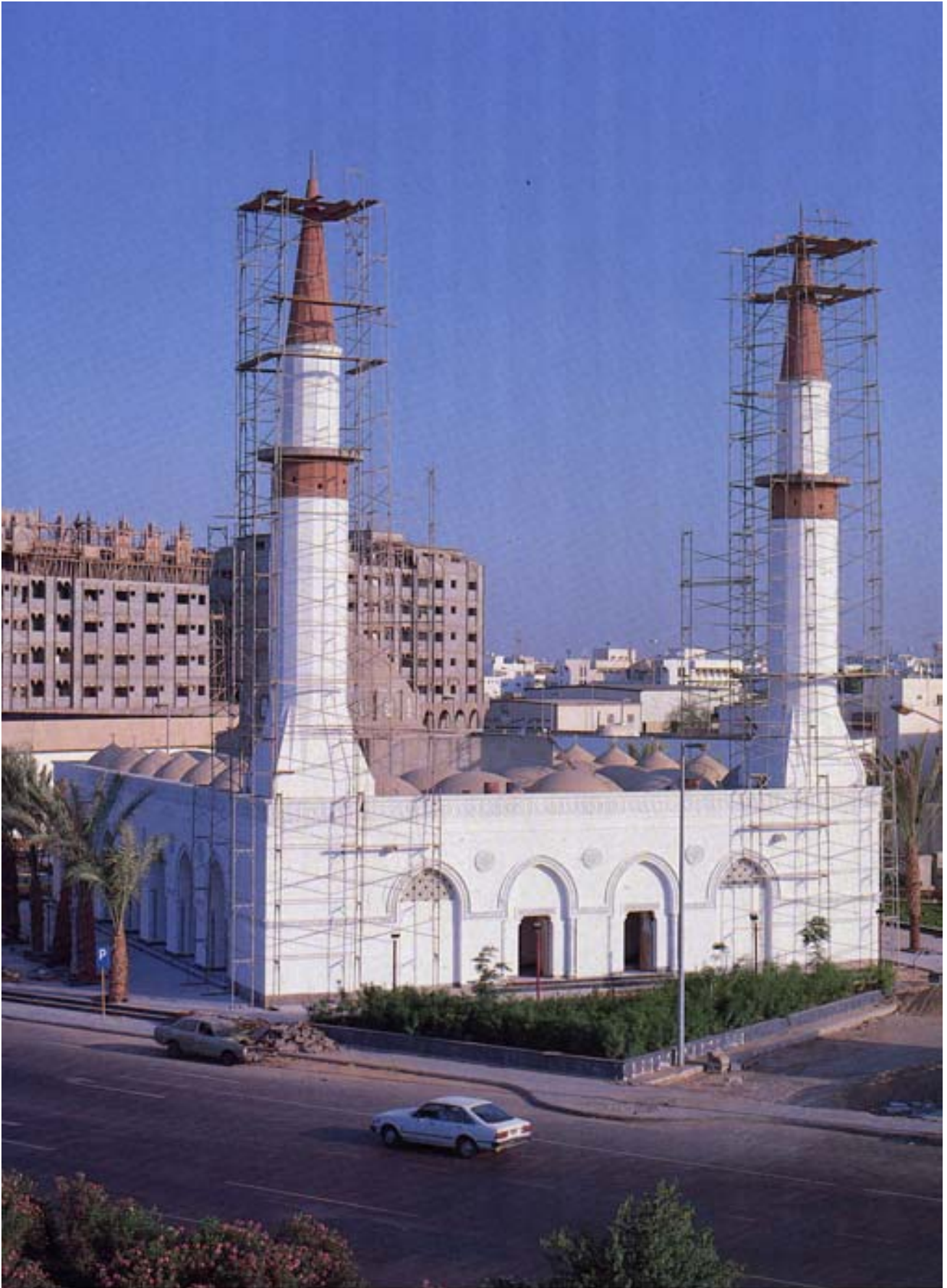
Harithy Mosque during Construction
