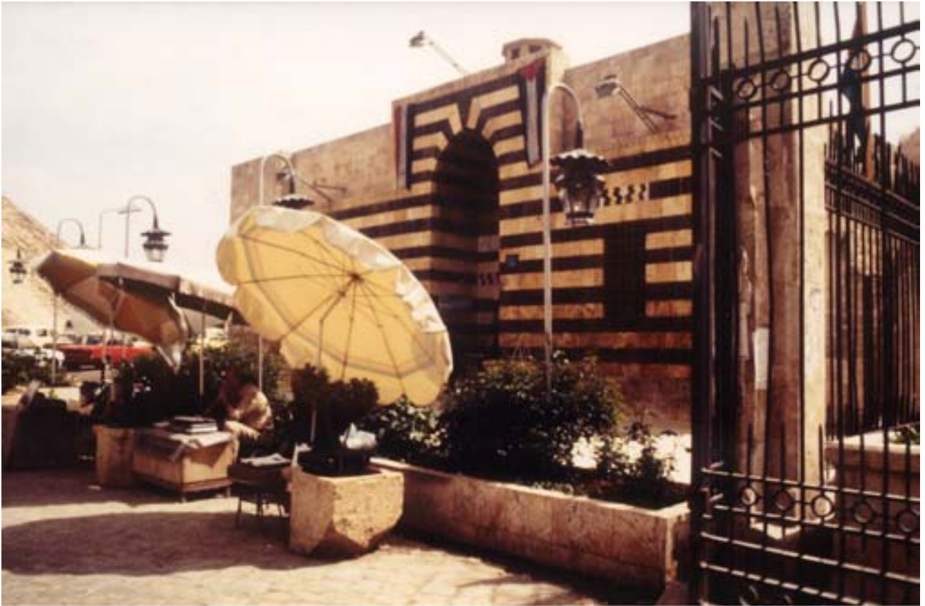
Entrance façade from south-west
