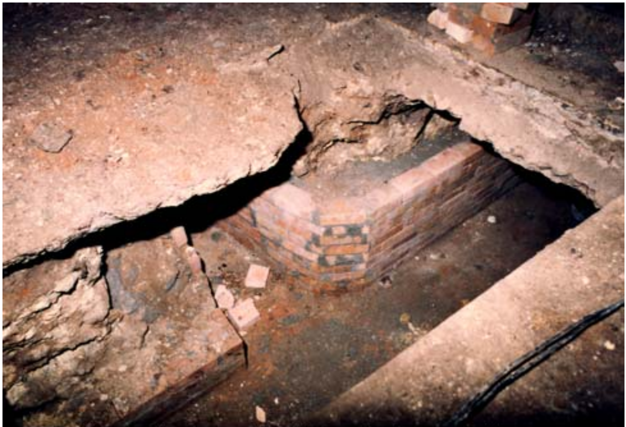
Al Qumim "heating room" and the tunnel underground wich warm the floor of Aljowani (interior part)
