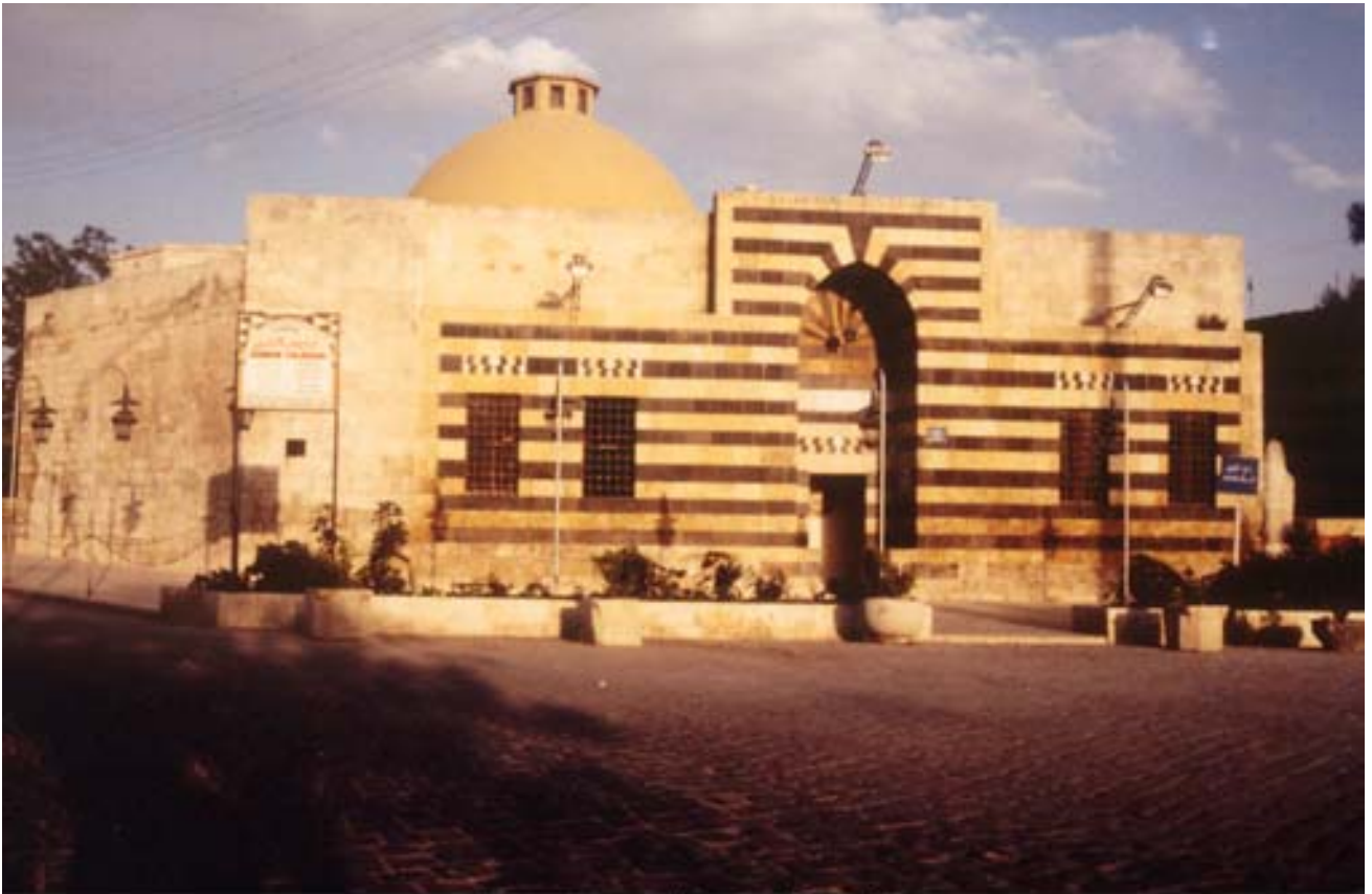
Hamman, entrance façade
