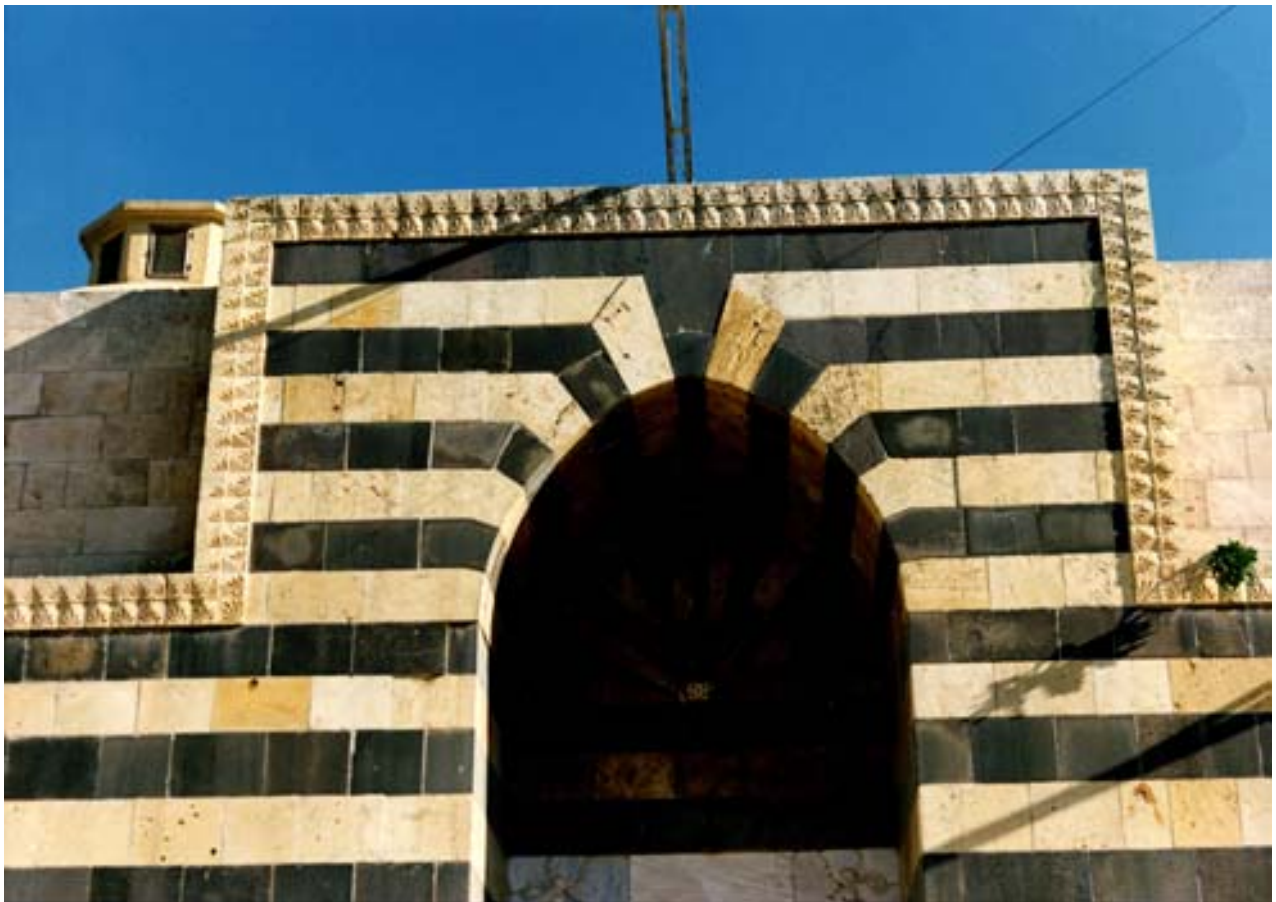
Detail of main Entrance
