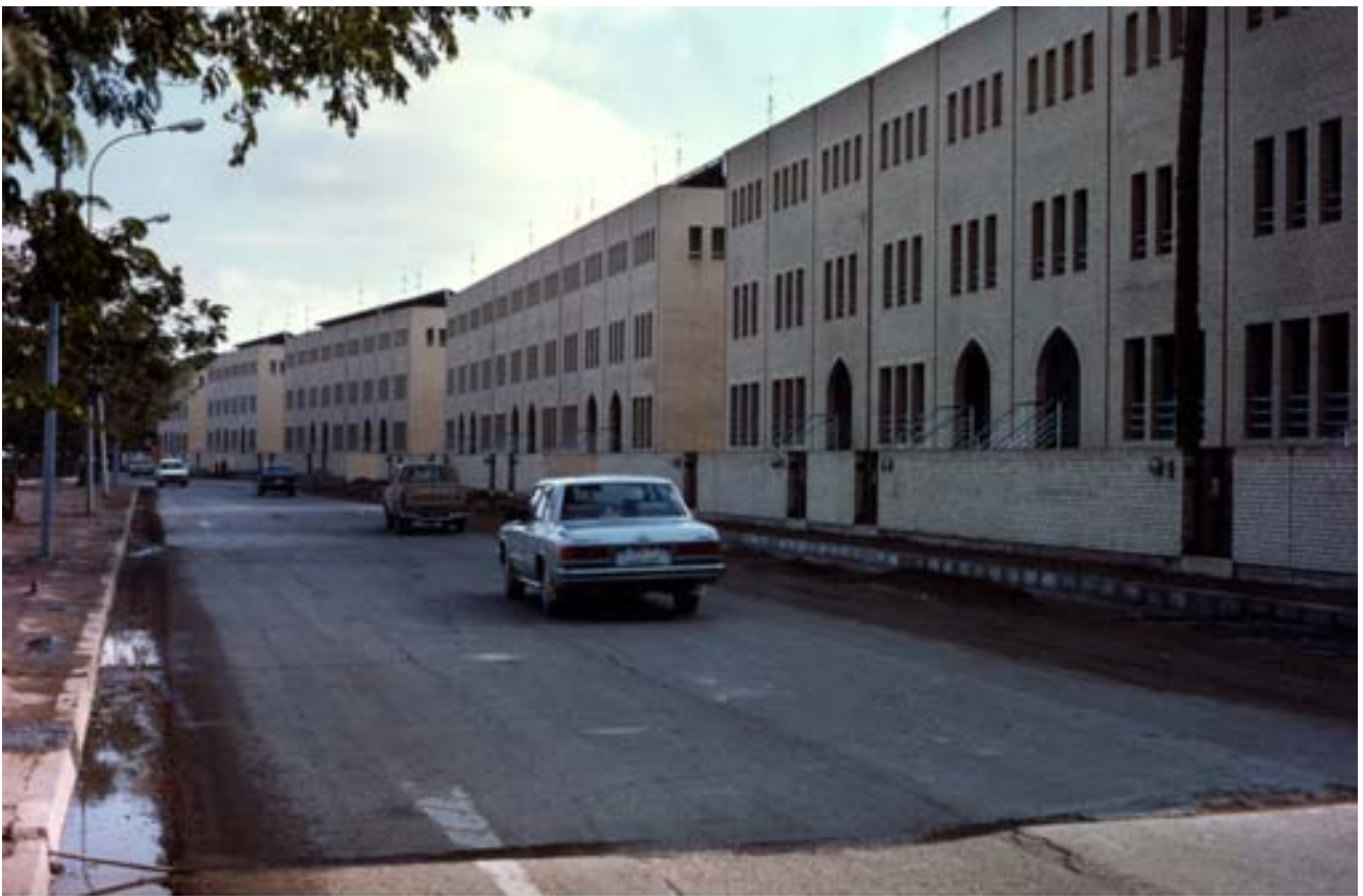
Front elevation along the street
