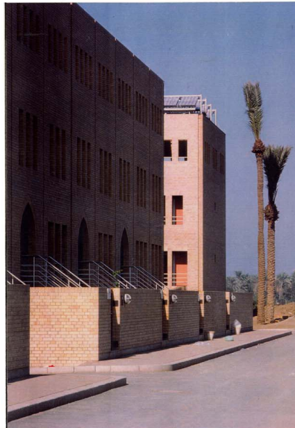
View along the main elevation
