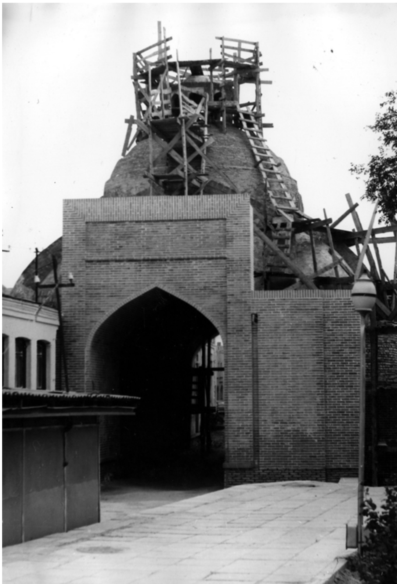
Tak-i Sarraphon, dome restoration work
