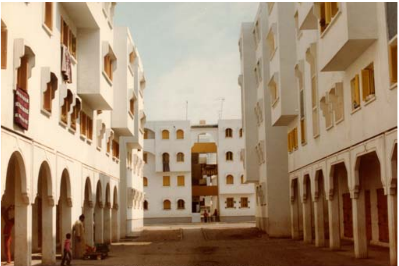
Pedestrian route bordered by shops
