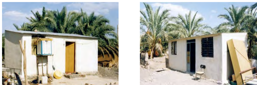
Figure 4: Units made of steel frame and masonry walls in the yard of destroyed houses (Source: Authors).
